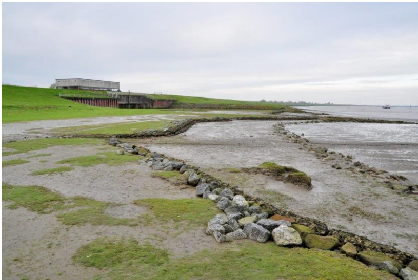
Protection of the erosion edge with rock rolls.
