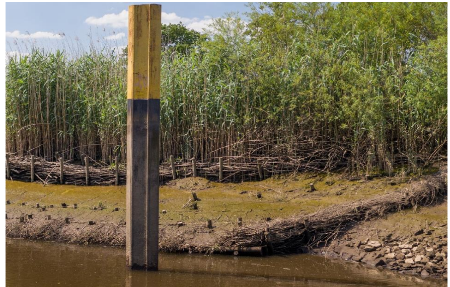
Test track 3 on the Wümme: brushwood box behind a pile wall (2014) and status of the adapted measure as of 2020 (right).
