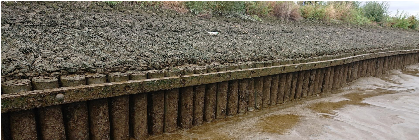
Pile wall toe protection and stone mattresses (on-site visit in October 2020).
