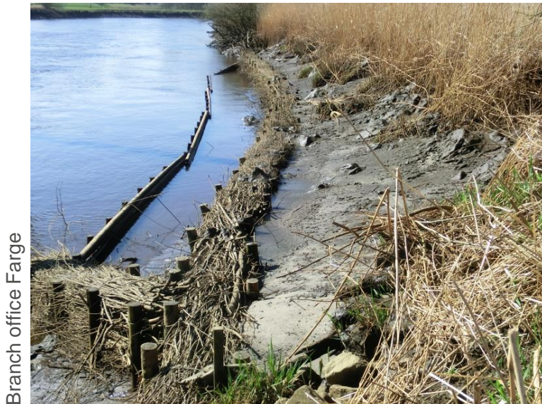
Test track 3 on the Wümme: brushwood box behind a pile wall (2014) and status of the adapted measure as of 2020 (right).
