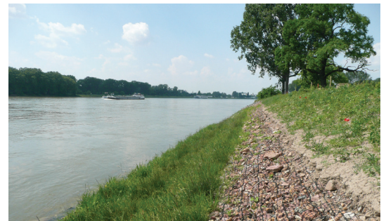
River Rhine, right bank, km 441,00 bis 441,05 (vegetation gabions and stone mattresses)
