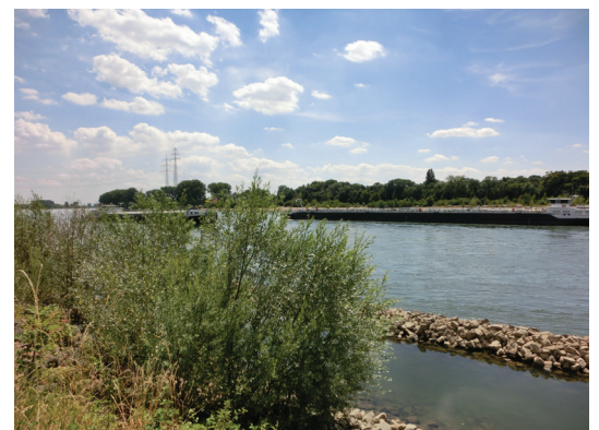
River Rhine, right bank, km 440,63 bis km 440,75 (vegetated riprap and stone wall with shallow water zone)
