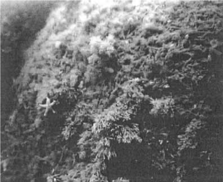
Figure 6. Sand bag surface with biological settlements
