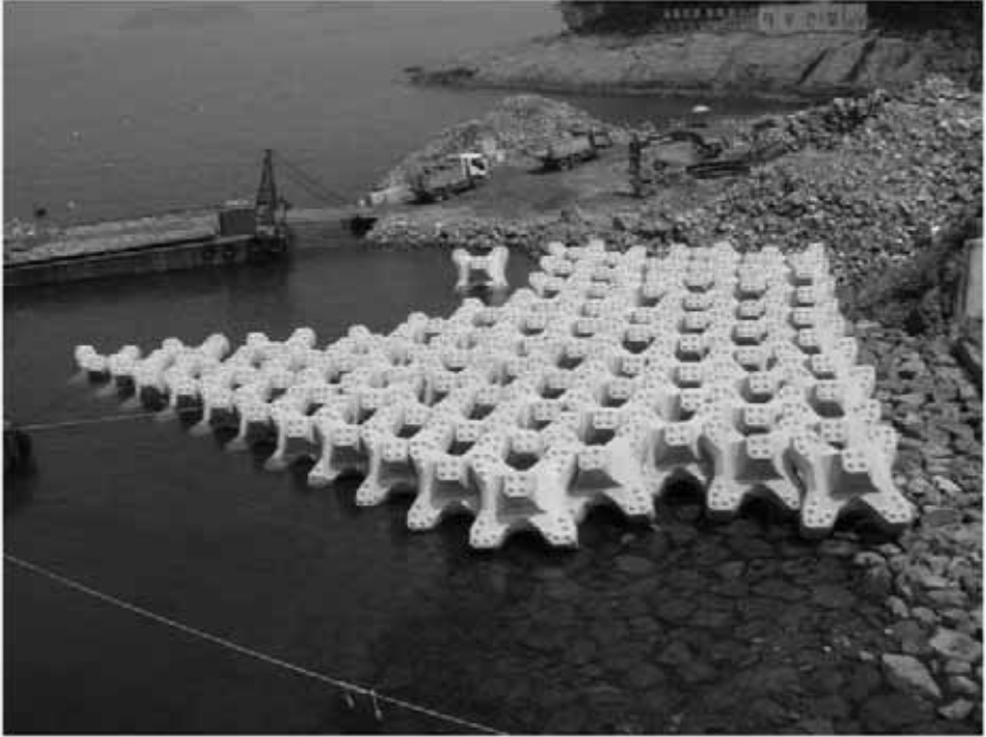
Figure 5. In situ systematic placement of ACCROPODE™ II units at the root of the structure.
