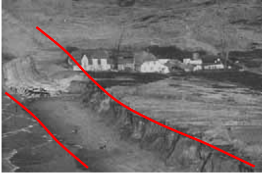
Figure 10: After storm surges in the year 2000, the second defense line is exposed to wave attack again since construction in 1990
