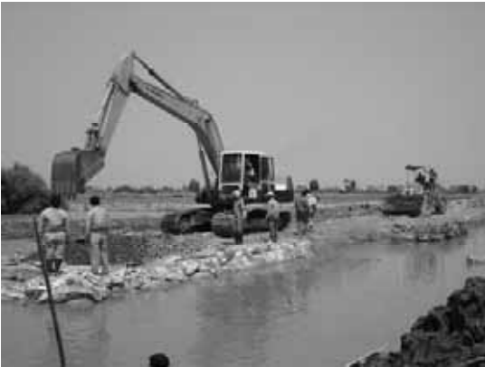
Figure 12: Installation of aggregate for access road on top of geotextile sand containers
