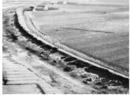
Figure 5. Deformations of the seaside slope at Friedrichskoog 1962 (Petersen/Rohde, 1991).
