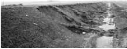
Figure 4. Sliding of the steep inner slope at Grothusenkoog 1976 (Petersen/Rohde, 1991).
