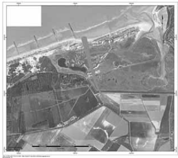
Figure 5. westward relocation of the entrance channel
