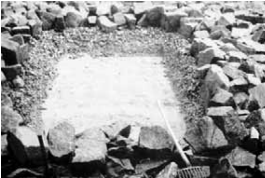
Figure 2. Nonwoven fabric after removing the revetment cover layers
