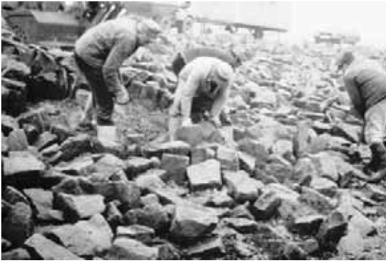
Figure 1. Digging out a filter fabric underneath rip rap of revetment
