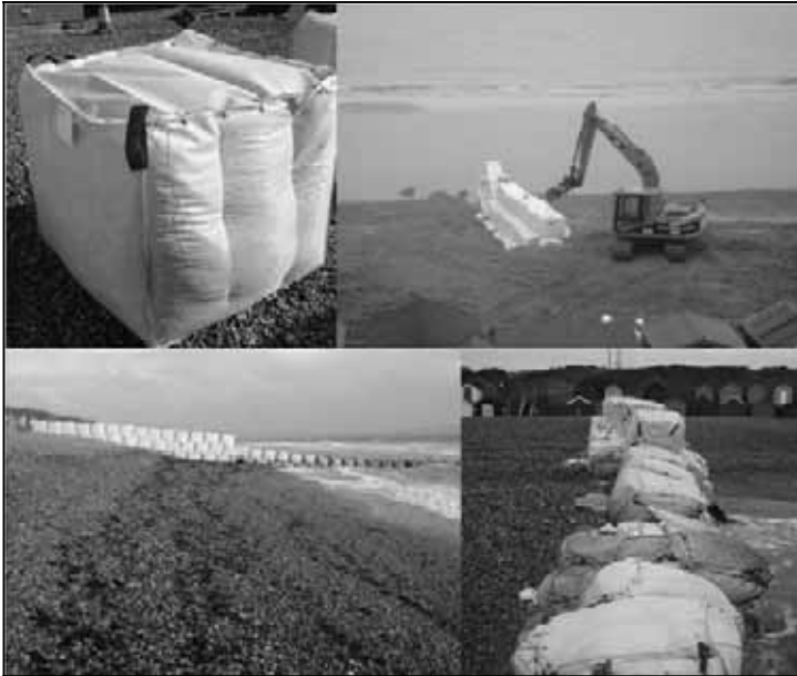
Figure 4. Top left: Geobag filled with beach material. Top right: view of structure from top of cliff. Bottom left: western elevation. Bottom right: view shorewards showing accretion-erosion across the structure with some damage evident.
