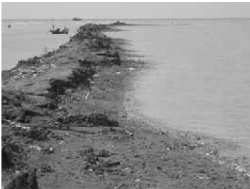
Figure 11: Old Jetty – heavily eroded
