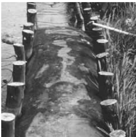
Figure 3. Sand filled tube in a land reclamation field
