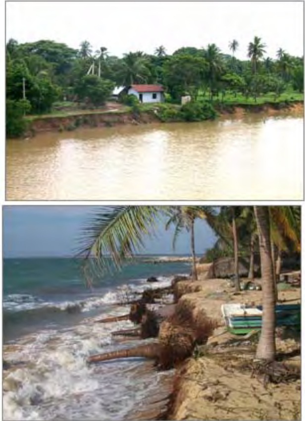
Figure 2. Illustrations from Sri Lanka: upper photo: river bank erosion, lower photo: coastal erosion at the southwest coast.
