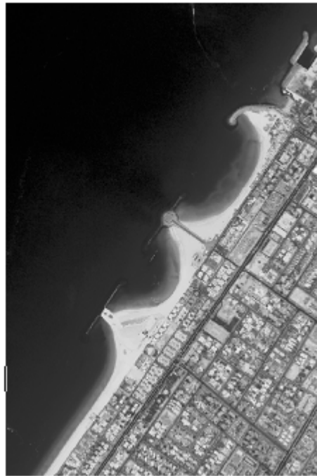
Figure 9. Shore parallel breakwaters and a small fishery port approx. 10 years after construction.
