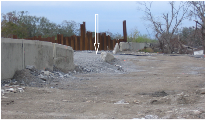
Figure 10. Piping failure in New Orleans
