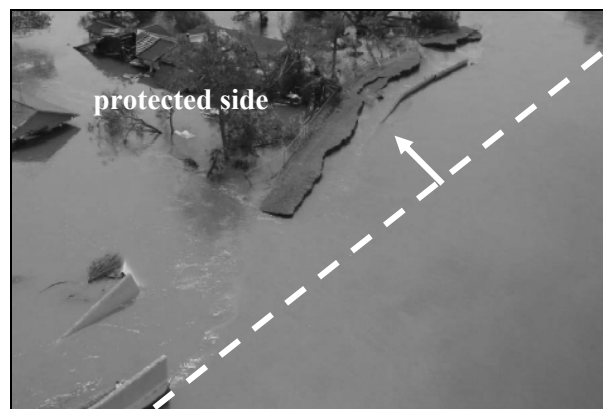
Figure 9. Stability failure in New Orleans due to hurricane Katrina (modified after ILIT, 2006)
