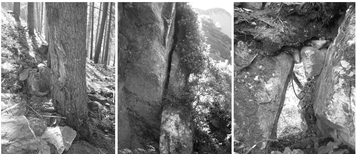
Figure 3. Examples of indicators. Left: Fresh damage of a tree caused by bouncing rock fragments (activity s.s.). Middle and right image: Wide open fractures, partly with stressed vegetation, indicating active loosening and instable conditions in the detachment zone.
