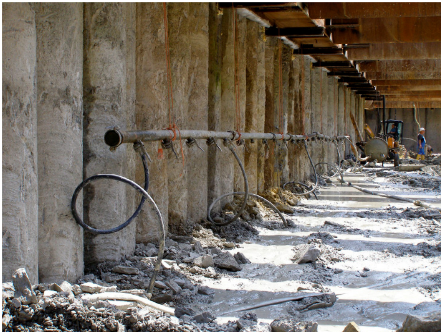
Figure 5. Relief wells installed to prevent hydraulic base failures at the bored pile wall
