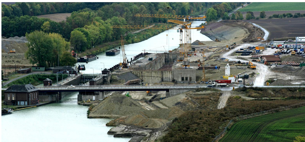
Figure 1. Construction site of the new ship lock in Bolzum
