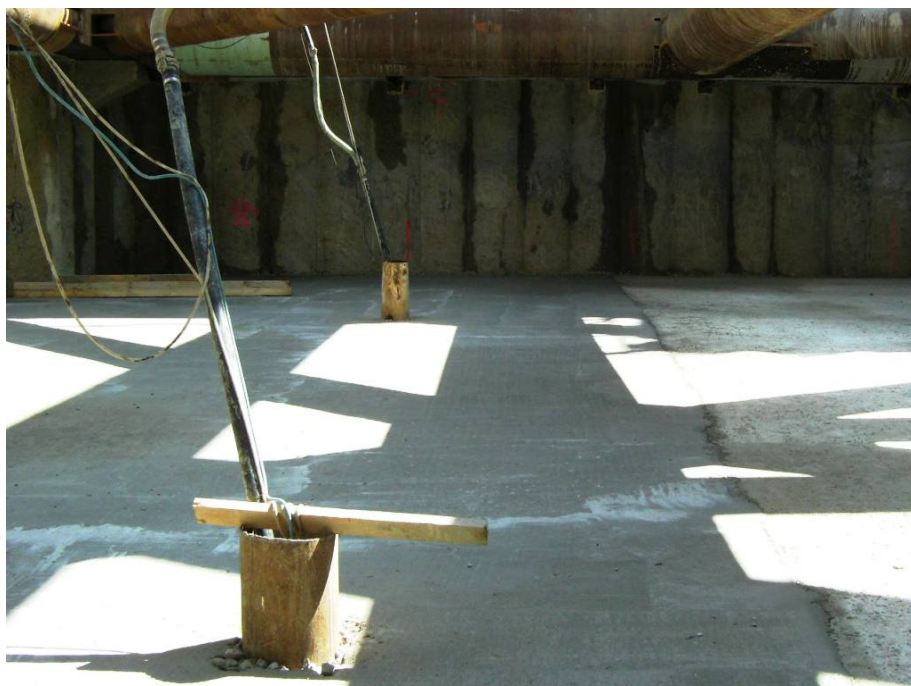
Figure 6. Relief well to prevent the bottom of the construction from uplift
