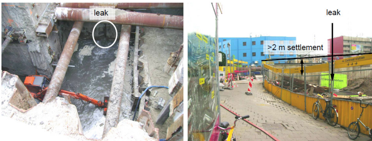
Figure 8. Photographs of leakage and ground surface settlement
