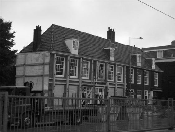
Figure 7. Subsidence along an underground station of the North-South Train Line in Amsterdam
