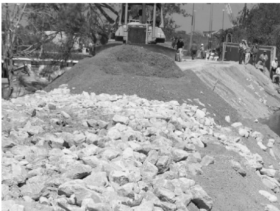
Figure 4. Creation of a new dike.
