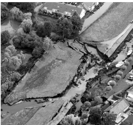
Figure 12. Failure of a peat dike in Wilnis
