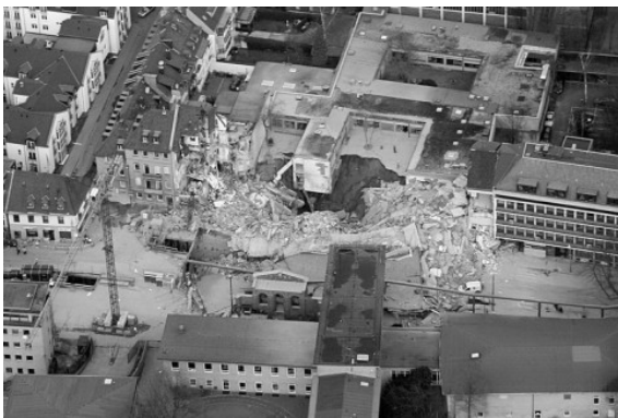
Figure 6. Collapse of a building pit of the North-South Line in Köln
