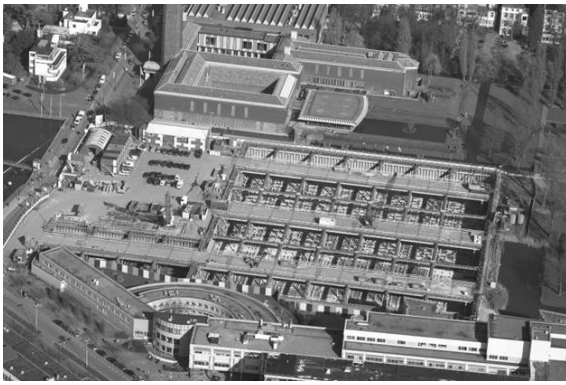
Figure 9. Construction of the Museum Park Garage in Rotterdam
