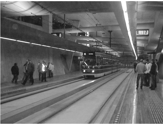
Figure 8. Big Market tram tunnel in Den Hague
