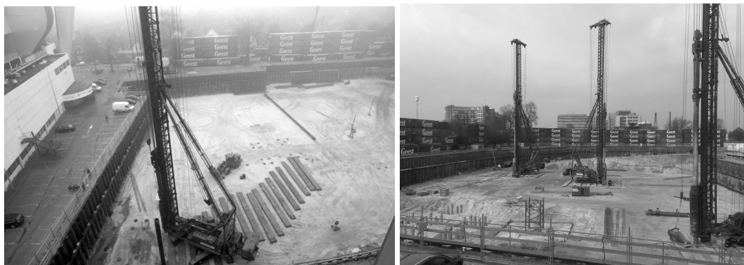
Figure 14. and Figure 15. Vibration and noise nuisance at precast pile driving in Eindhoven
