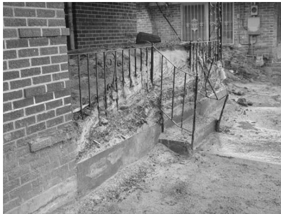
Figure 3. Thickness of the washed-in sand layer.
