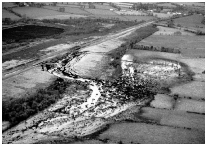
Figure 13. Failure of a peat dike in Edenderry
