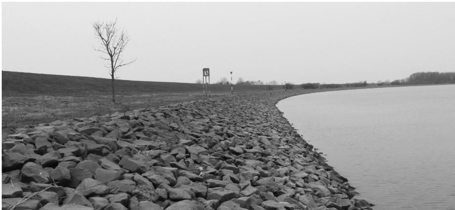
Figure 1. Rip-rap on the banks of Ems River (Germany) as a protective layer to prevent erosion of bank slope by hydraulic loads.
