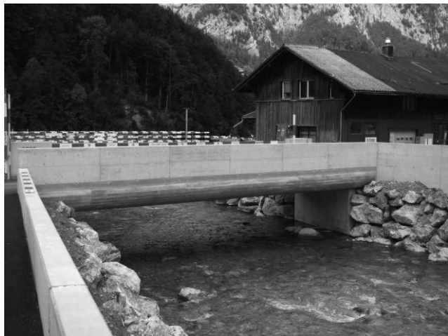
Figure 9. New baffle bridge at River Chirel, Switzerland
