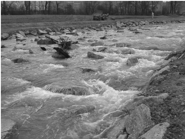
Figure 5. Ramp type B with unstructured blocks at the Wyna River (Canton Aargau, Switzerland) with a specific discharge q of about 0.16 \text{ m}^2/\text{s} (view against flow direction). Source: Hunziker Zarn & Partner.
