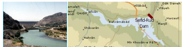
Figure 1. The Sefid-Rood Dam at the intersection of two rivers.
