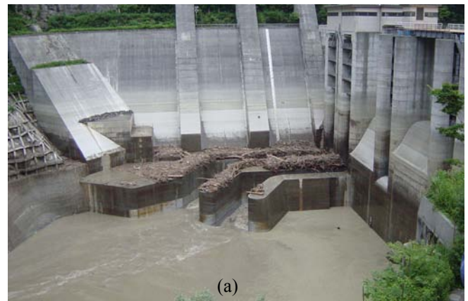
Figure 4. (a) Photo of Dashidaira dam during draw down flushing; (b) Plan view of Dashidaira reservoir topographic map
