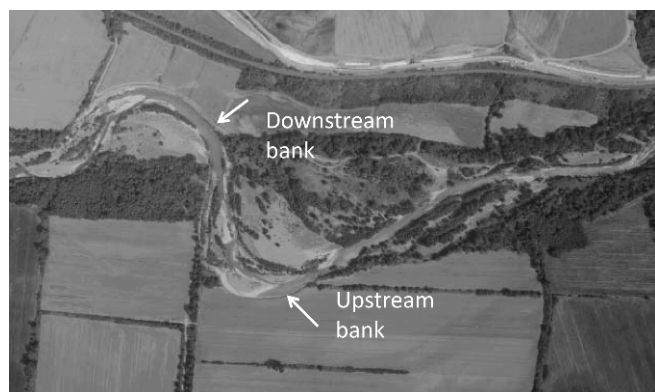
Figure 2. 2006 aerial photograph showing the study reach and monitored bank (aerial photograph reproduced by permission of Provincia di Pisa).
