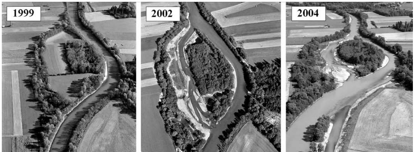
Figure 4. Bank retreat after initiation of a new side arm within a restored section at Kleblach-Lind at the Drava River (source: Carinthian government).
