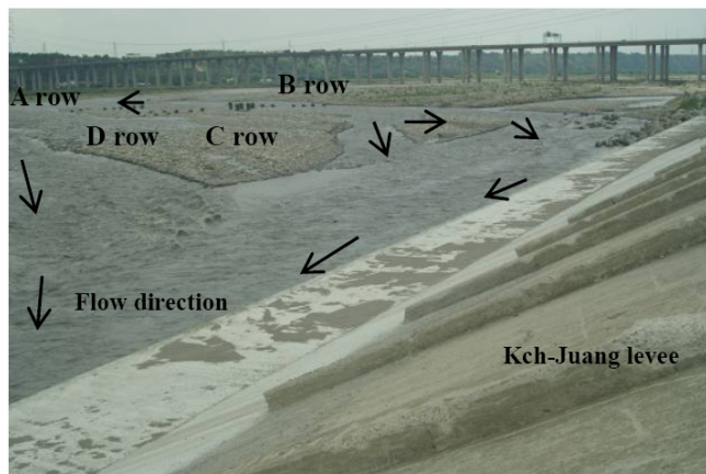
Figure 12 Low flow after plum rain finished on June 15th, 2007
