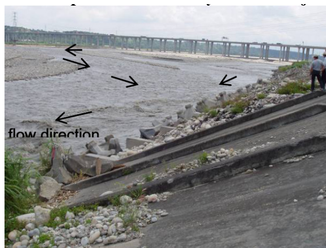
Figure 3 Two flows meet at the left bank levee-protection site
