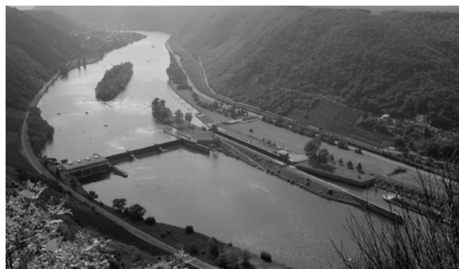
Figure 1. Barrage Lehmen with power plant, weir and ship lock at federal waterway Mosel
