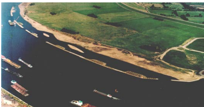
Figure 2: Longitudinal dam in the Rhine river at Bruckhausen (Duisburg), Germany.
