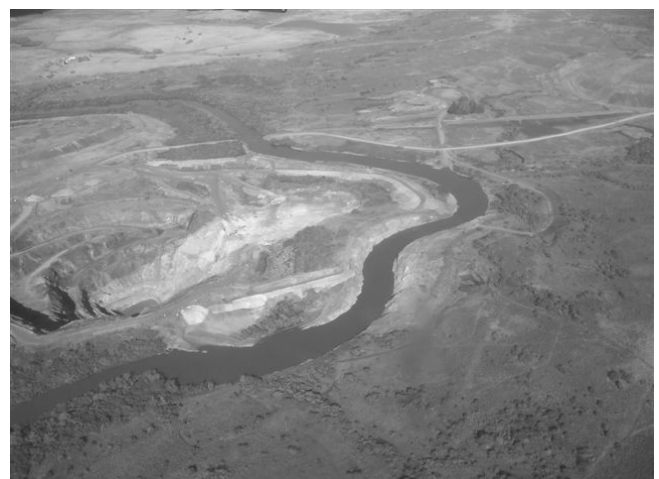
Figure 20. Aerial view during the flood of October 2007.
