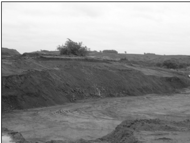
Figure 23. Upstream zone of the channel after construction
