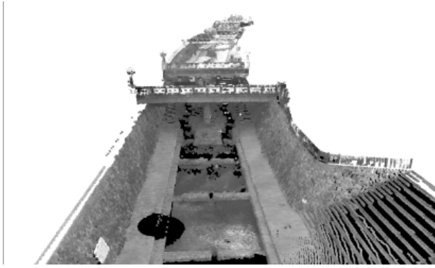
Figure 9. Measurement data by ground laser instrument
