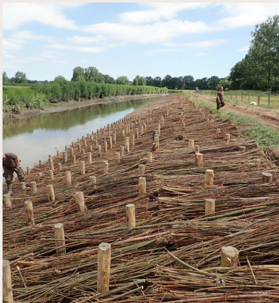
Brushwood mattress to protect dike without foreland (WSA Weser-Jade-Nordsee)
