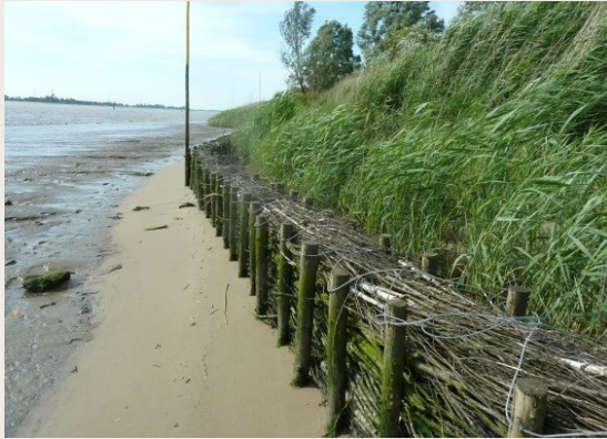
Brushwood box for stabilising an erosion edge (WSA Weser-Jade-Nordsee)
