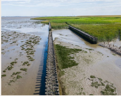
Double pile rows with stone filling and openings in offset arrangement (BAW)
