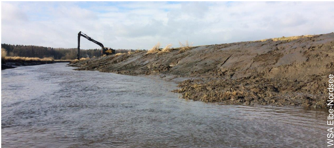
Reprofiling work in 2019.
