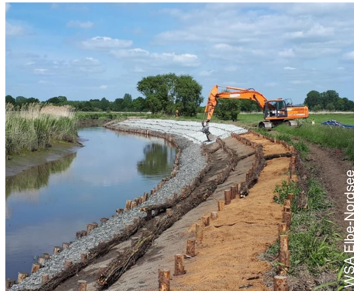
Construction of the measure in 2020.
