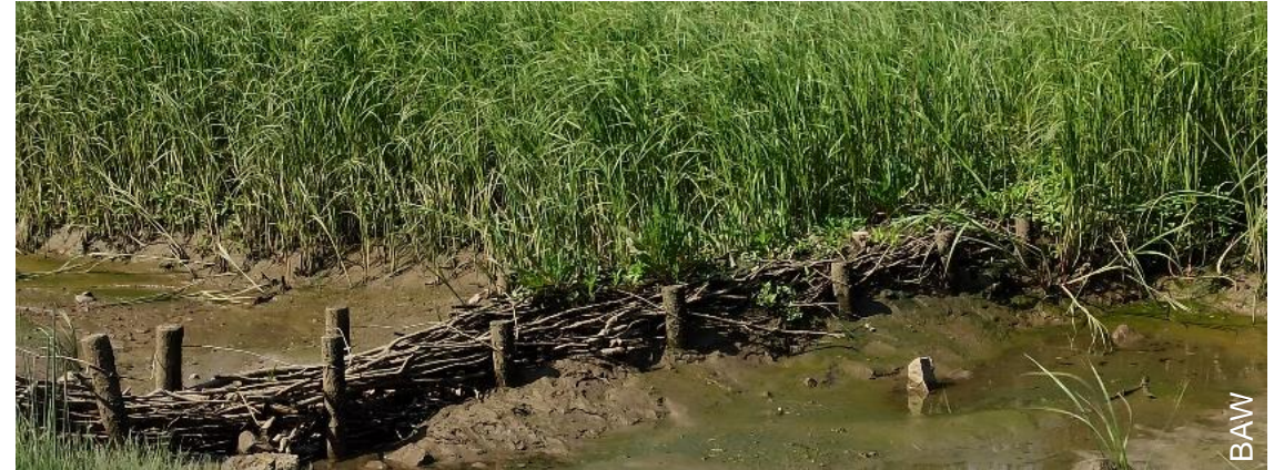
Brushwood box before maintenance in June 2023 .
