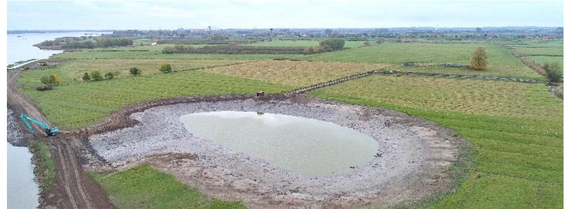
Riparian inlet during construction in 2020
