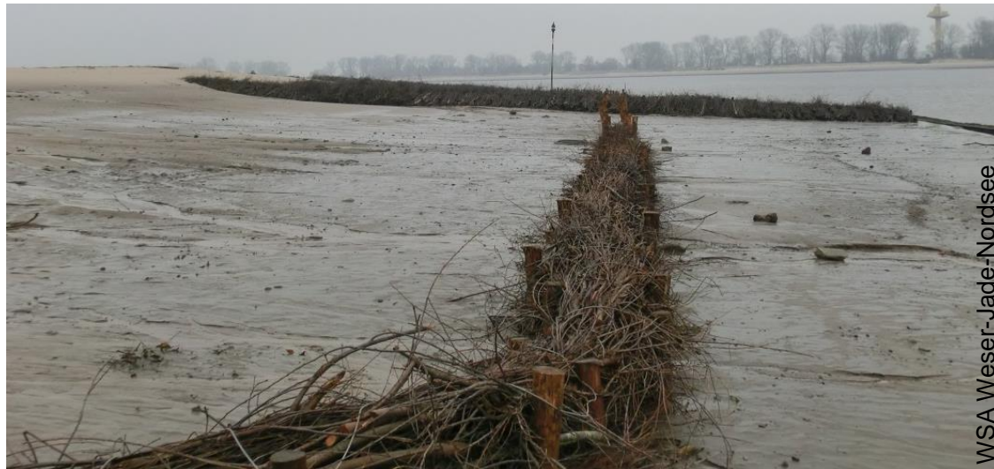
Brushwood training wall during construction in 2013.
