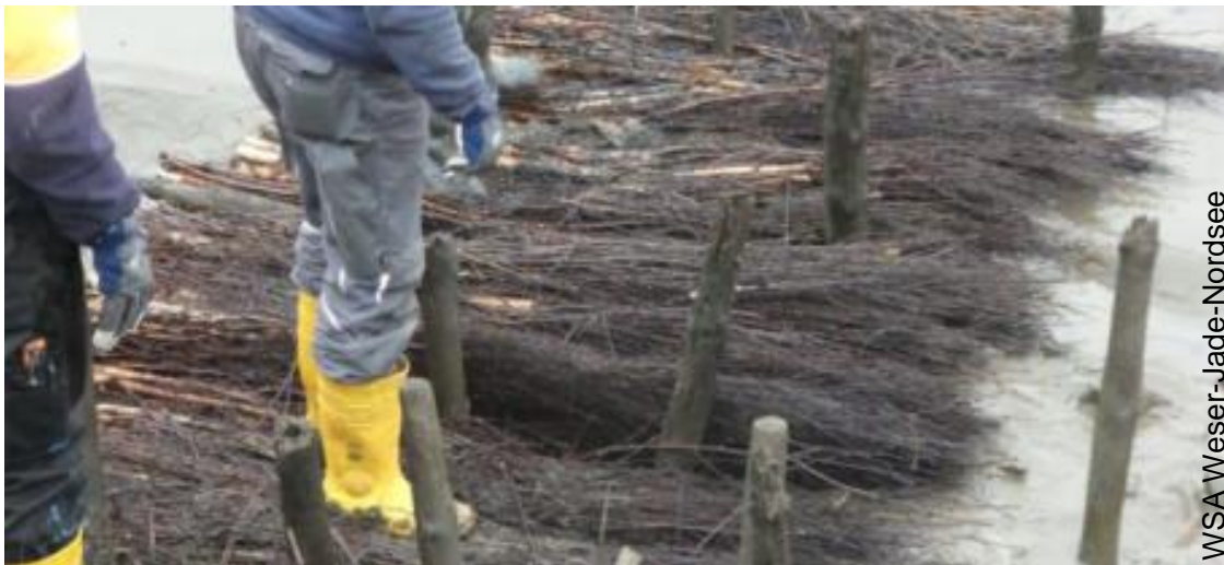
Construction of the measure in 2023
