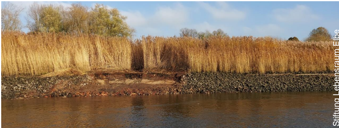
After lowering of the revetment.
