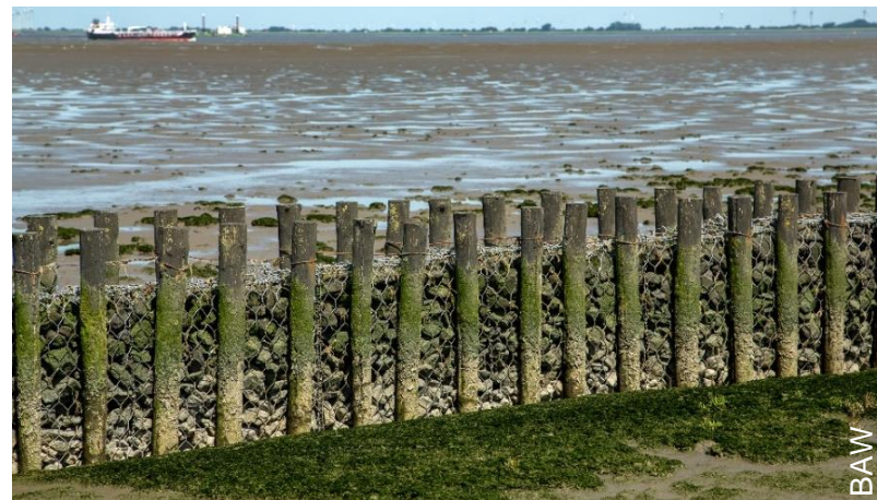
Protection of the erosion edge with a brushwood mattress in 2020.
