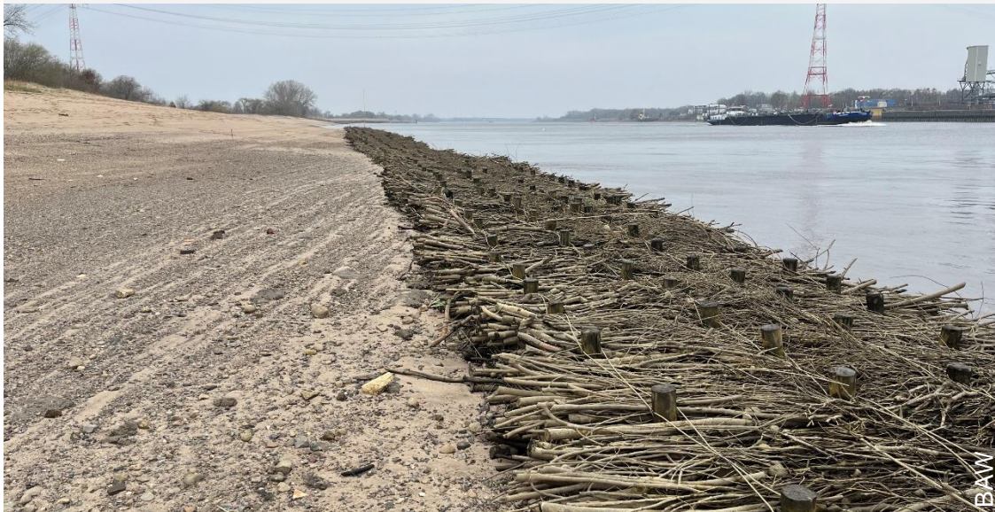
Brushwood training wall in section 2 at km 25,45-25,95 in March 2026.
