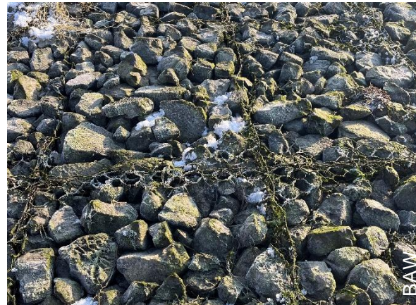
Beginning break down of the wire mesh (01/2026).
