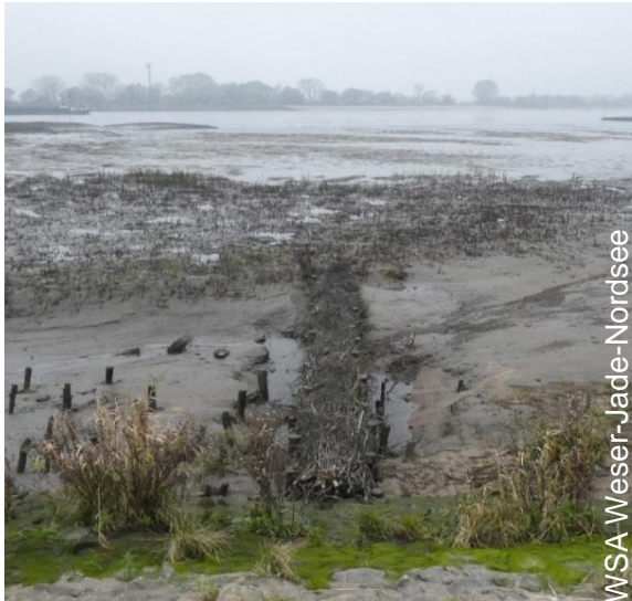
Brushwood box after construction in November 2020.
