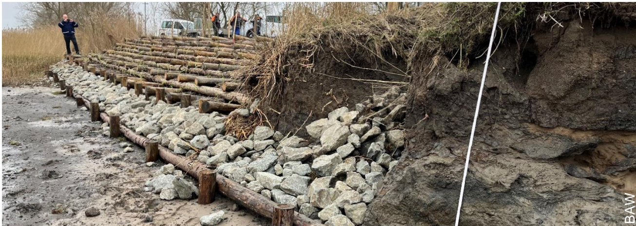
Finished crib wall with initial plantings in March 2026.
