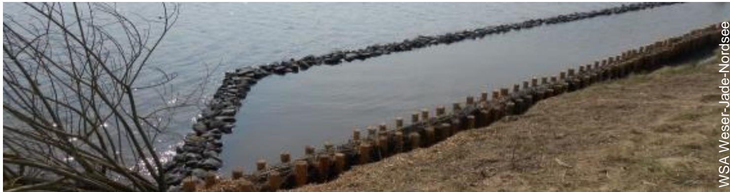
Finished measure immediately after construction in 2018.
