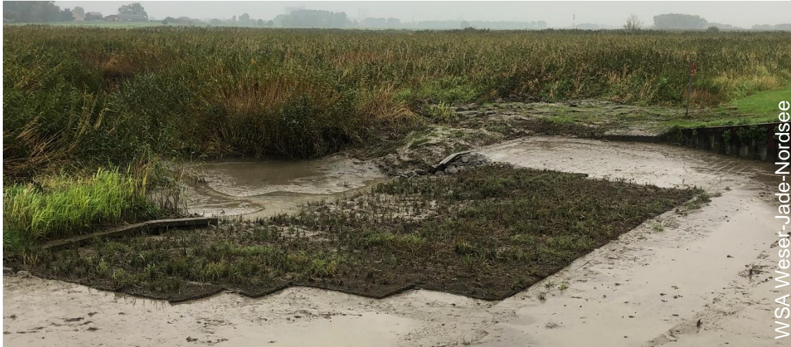
Measure immediately after construction (08.10.2020)
