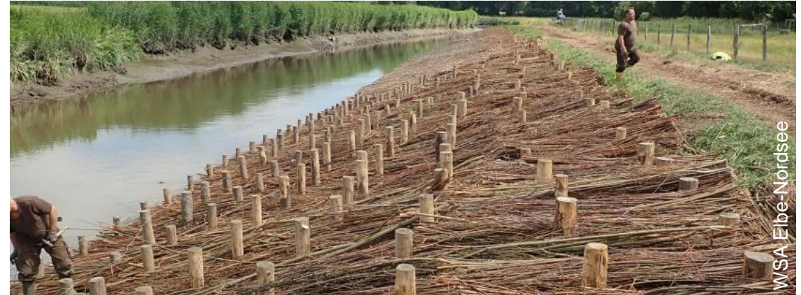
Measure during construction in 2018.
