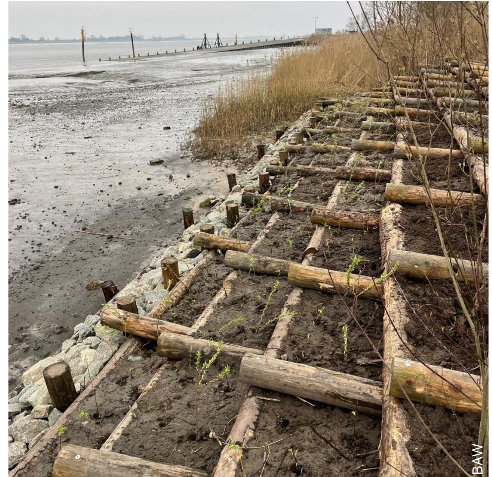
Finished crib wall with initial plantings in March 2026.
