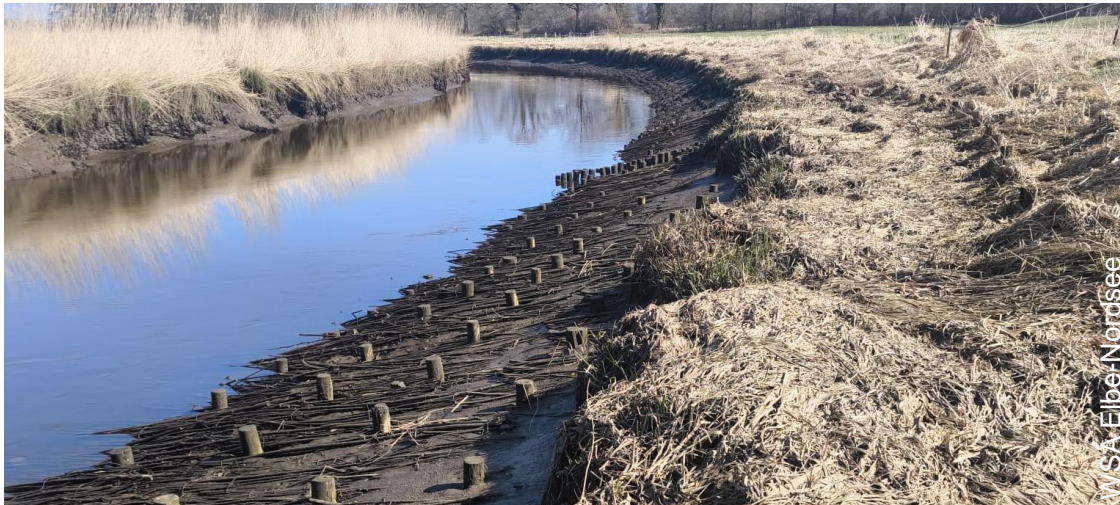
Measure in April 2026, upper part covered by vegetation.
