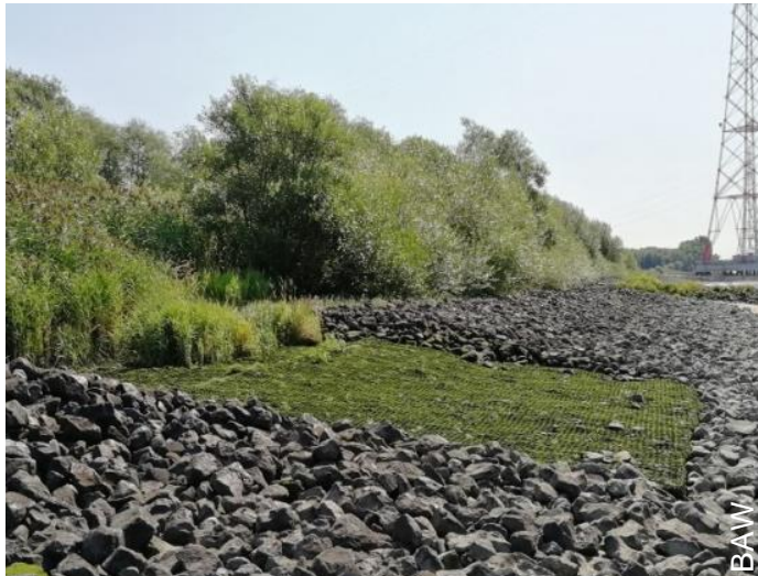
Beginning break down of the wire mesh (01/2026).
