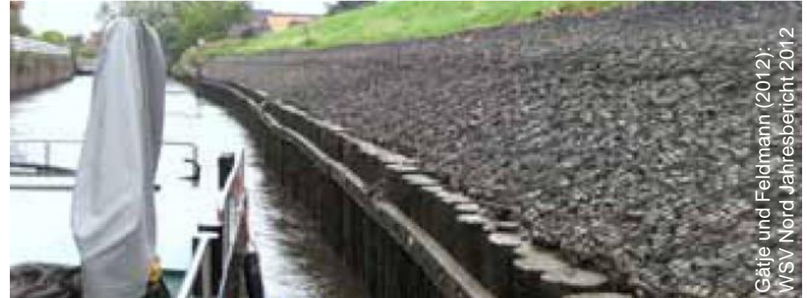
Implemented measure with pile wall toe protection in 2012
