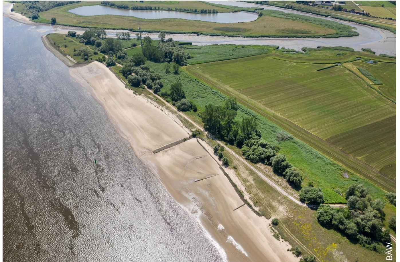
Brushwood mattress for bank protection placed at the height of the groyne root.
