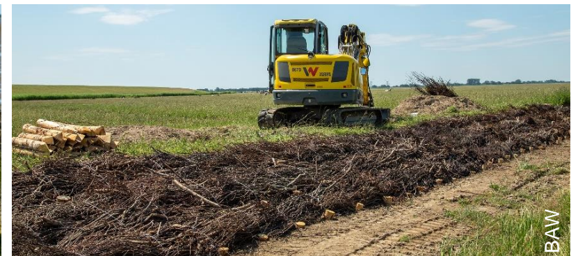
Protection of the erosion edge with a brushwood mattress in 2020.
