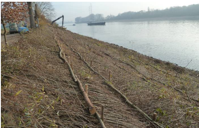
Figure 2: Construction of willow brush mattresses (perpendicular to the direction of flow)
