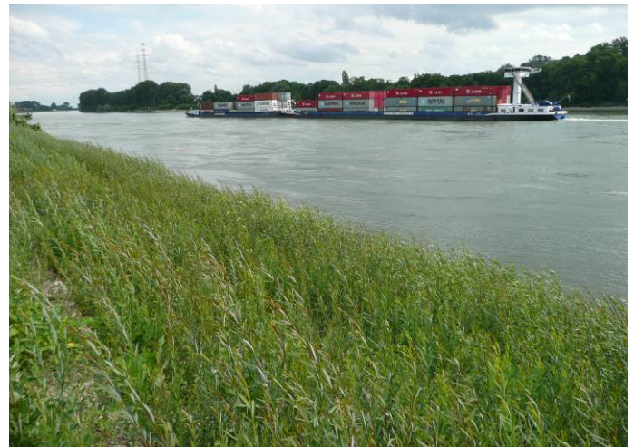
Figure 7: Growth of willow-brush mattresses (six months after construction)
