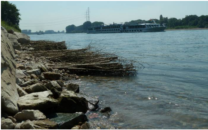
Figure 5: (Dead) wood fascines at low-flow water level
