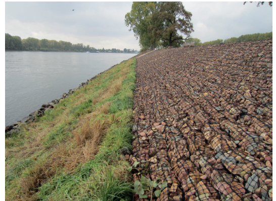
River Rhine, right bank, km 441.000 - km 441.110 (reed gabions, stone mattresses)
