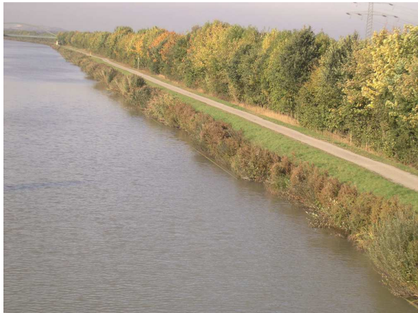
Figure 2: Rapid establishment of vegetation on the bank protection on the MLK, using alginate-enriched topsoil
