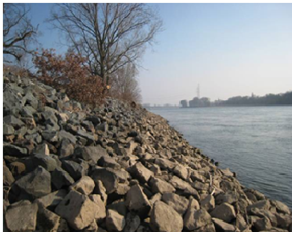
Figure 2: Old riprap revetment; picture taken on 22 February 2011
