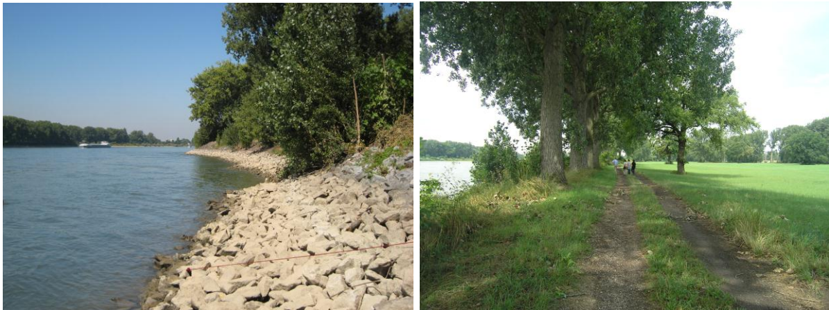
Figure 2: The test stretch today; (left) riprap with brushwood; (right) poplars at the top of the slope and maintenance path
