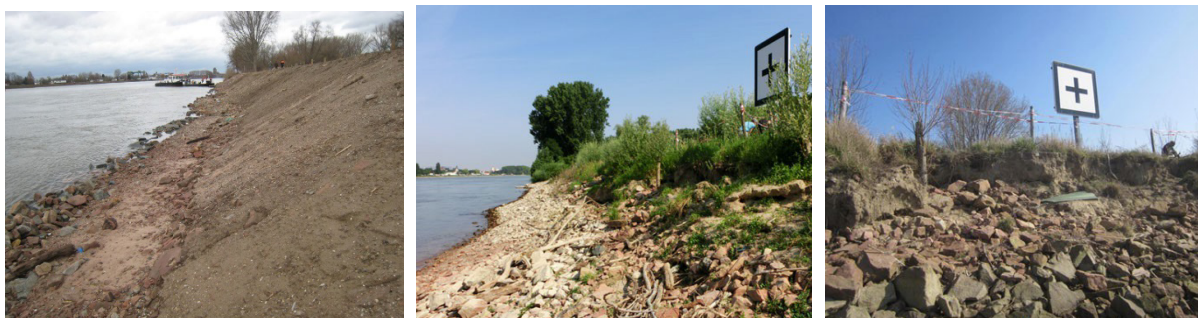
Figure 35: Development in TF 9 – 12/2011 (left, after completion of construction), 7/2013 (centre), 3/2014 (right) (photo: BAW)
