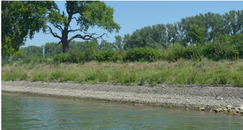
Figure 20: TF 5b – Stone mattresses, well vegetated on the upper half of the slope and with almost no vegetation on the lower half (2.7.2015) (photo: BAW)
