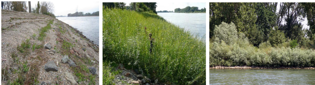
Figure 9: Overview: development of willow brush mattresses in TF 3 – 4/2012 (left), 7/2012 (centre), 7/2017 (right) (photos: BAW)
