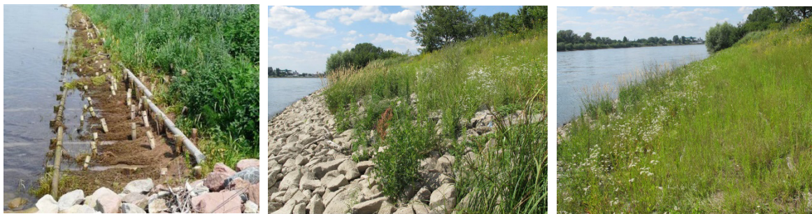
Figure 22: Damage in the lower slope area 5/2012 (left); rehabilitated condition 7/2017 (centre); good development in the upper slope area (right) 7/2017 (photos: BAW)
