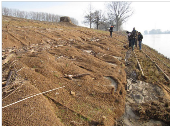
Figure 27: Slope deformations after flooding in TF 7a, upper zone (22.3.2012) (photo: BAW)
