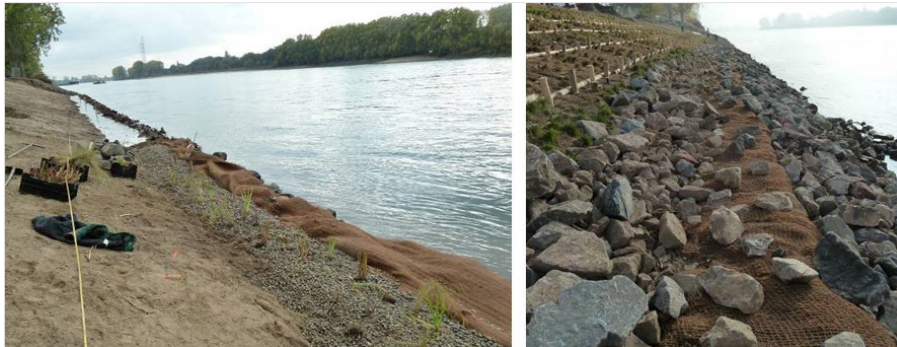
Figure 29: Reed rolls during and after installation in 2011 (photos: Katja Behrendt/ Hans-Werner Herz, BfG)
