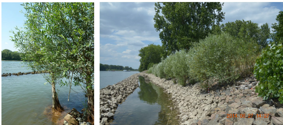
Figure 30: Left: willow branch cutting with adventitious roots (07/2013); right: vigorous development of willow plantings (06/2014) (photos: Katja Behrendt/Hans-Werner Herz, BfG)
