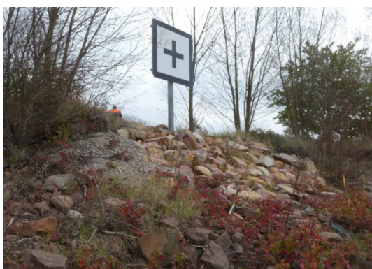
Figure 39: Km-sign at km 441.500 secured with armourstones (7.11.2017) (photo: BAW)
