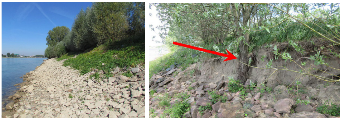
Figure 37: Left: old armourstones in the ground exposed by water in TF 9 (8.9.2016); right: log branch cuttings exposed by water (26.04.2018) (photos: BAW)
