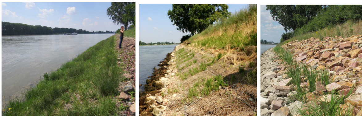
Figure 17: Development of the gabions, from left: 07/2012 – 07/2013 – 07/2017 (condition rehabilitated with one stone layer) (photos: BAW)
