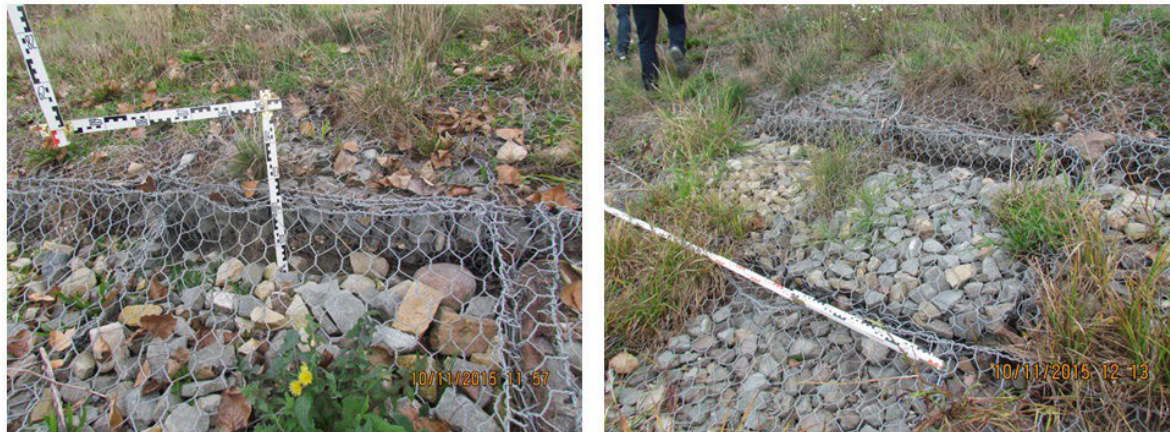
Figure 18: Reed gabions on 10.11.2015, vertical edge due to stone displacements within the gabions (photos: BAW)
