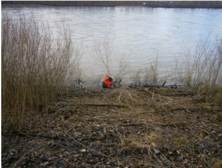
Figure 64: Partial pruning of the willow brush mattress in TF 3 (January 2015) (photo: WSA Upper Rhine)
