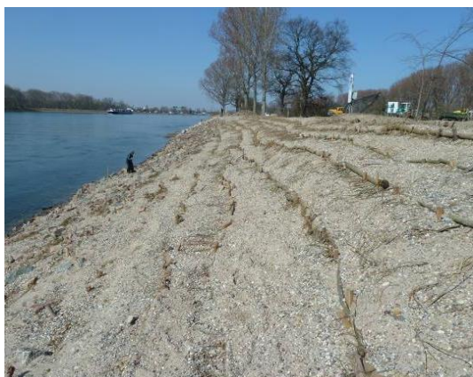
(7) Sand-gravel blend covering willow brush mattresses; Dec. 2011
