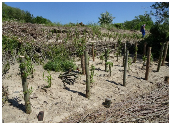
Figure 3: Typical maintenance work for live willow mats. Left: Cutting of branches. Right: Planting of willow stakes after storm event. Source: WSV.
