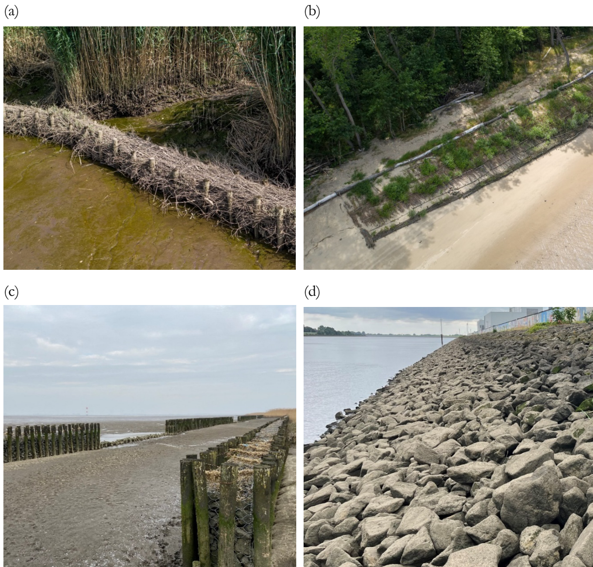
Figure 1: Nature-based solutions for bank protection in German estuaries, brushwood box (a), live willow mat (b), gabion box (c), and in comparison, hard-engineered bank protection, rock armour revetment (d). Source: BAW.
