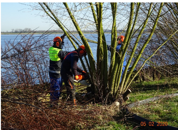
Figure 3: Typical maintenance work for live willow mats. Left: Cutting of branches. Right: Planting of willow stakes after storm event. Source: WSV.
