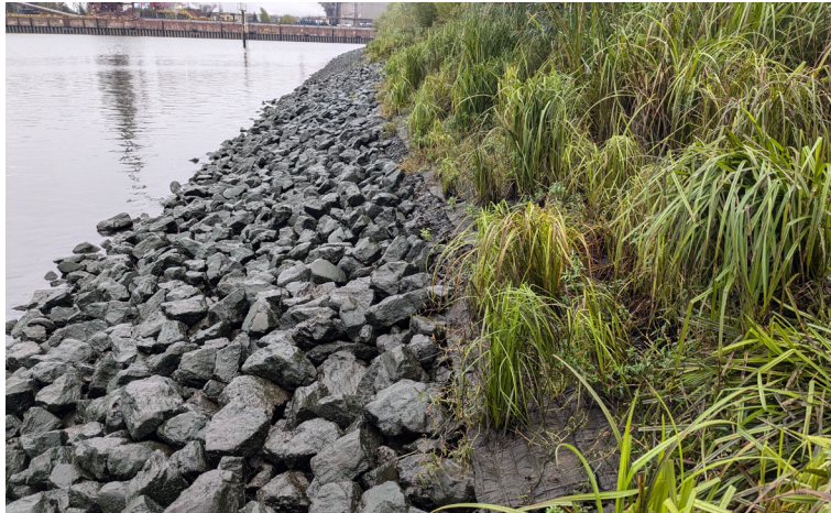
Figure 12: Vegetated riprap using pre-vegetated mats at the Elbe (picture source: BAW).
