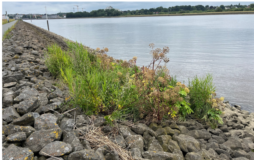
Figure 11: Integration of vegetation into existing riprap revetments along the Lower Weser (picture source: BAW).
