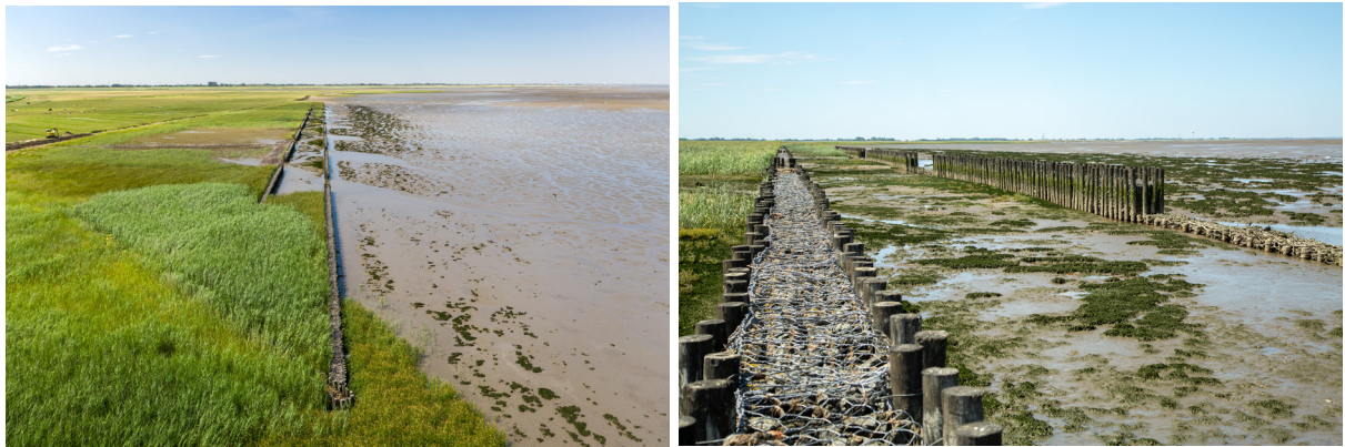
Figure 8: Example of an indirect bank protection with regular openings in the Elbe estuary consisting of two double pile rows with gabion filling and regular openings (picture source: BAW).
