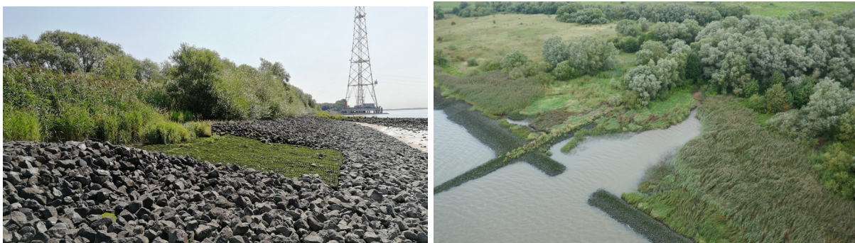
Figure 10: Examples of a lowered revetment on the River Elbe, allowing for vegetation development (left) and increased tidal exchange (right) (picture source: BAW).
