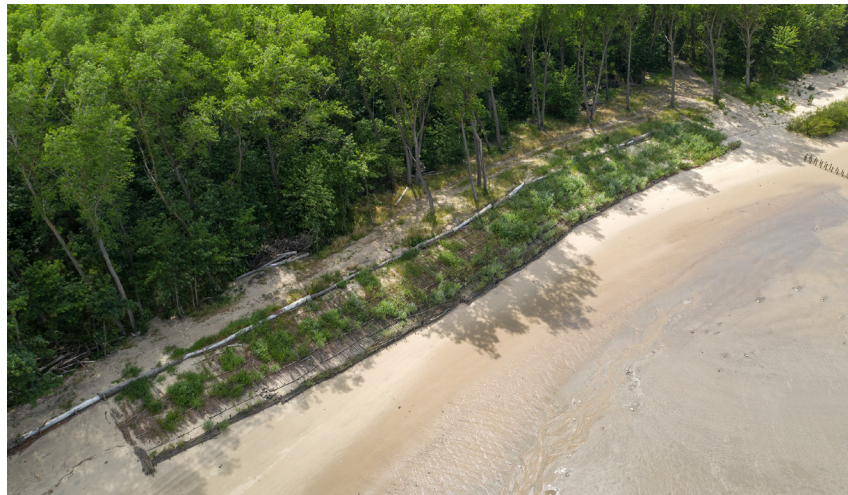
Figure 9: Living willow mattress for beach protection at the river island Hanskalbsand at the Elbe (picture source: BAW).
