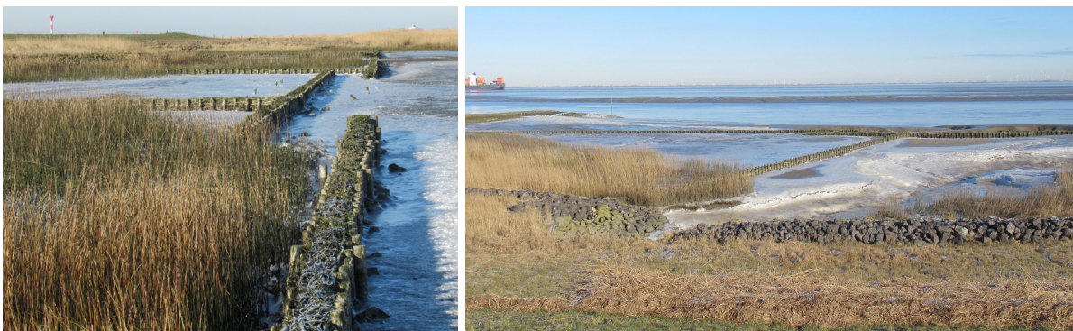
Figure 7: Brushwood boxes for bank protection within a groyne field on the Oste near its entrance into the Elbe. (picture source: WSA Elbe-Nordsee).
