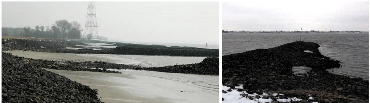
Figure 3: Characteristic damage to groynes at Juelssand (Lower Elbe Estuary) caused by long-period ship wave action. Destruction of the groyne root (left) and erosion of the crest and lee side slope (right).
