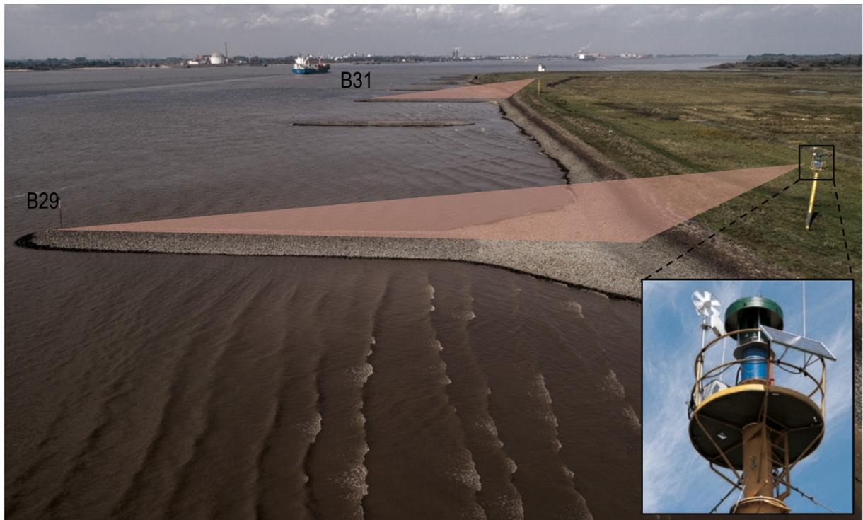
Figure 10: Set-up for monitoring of groyne topography at low tide levels with pile-mounted laser scanners. Close-up of the monitoring platform with laser scanner housing.
