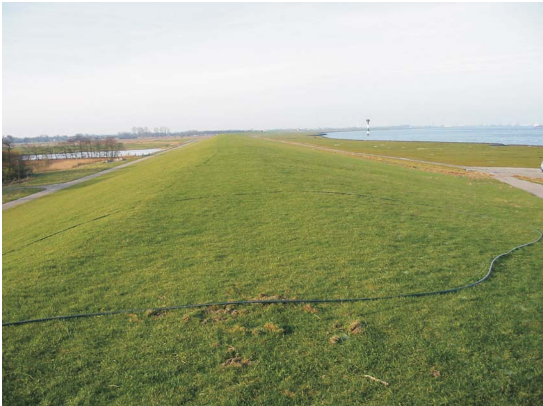
Fig. 5.15: Dike covered by grass (photo: SCHÜTTRUMPF)
