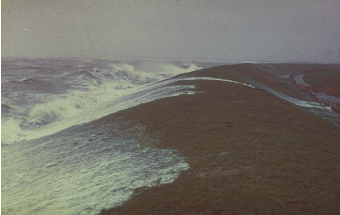
Fig. 5.23: Short crested waves resulting in wave run-up and wave overtopping (photo: ZITSCHER)
