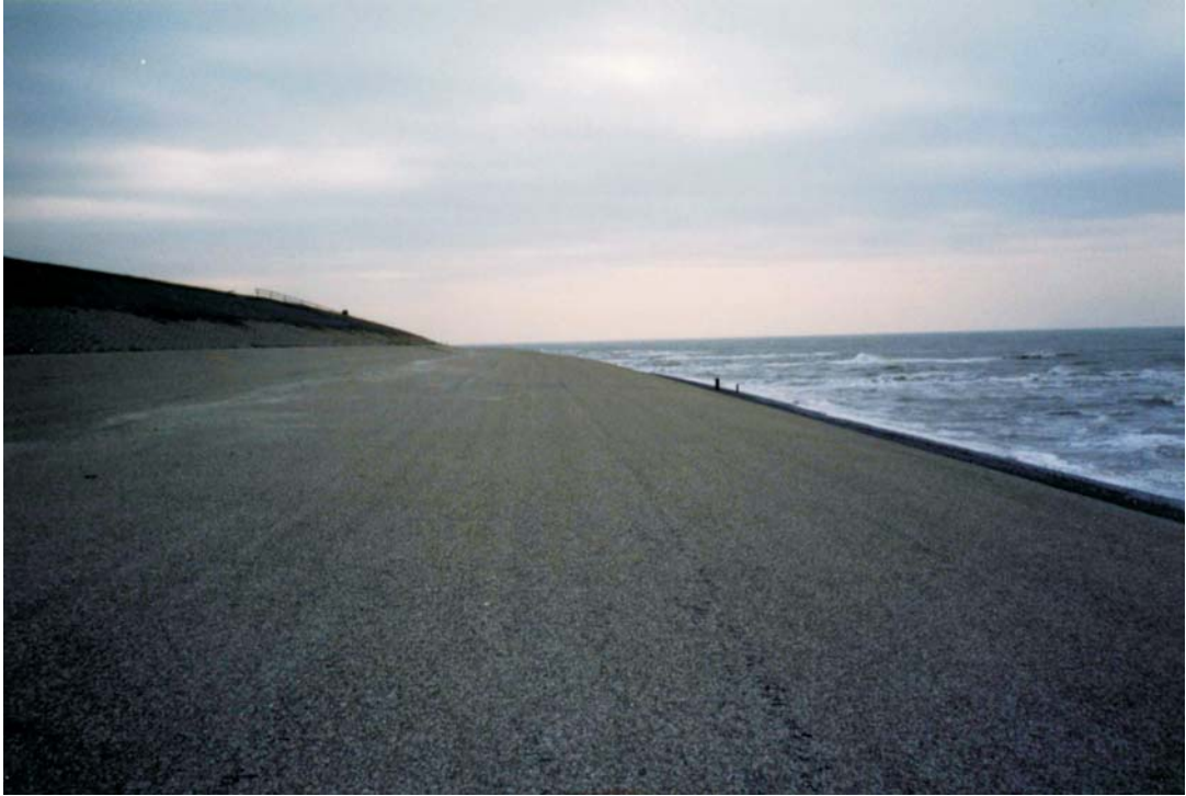
Fig. 5.16: Dike covered by asphalt (photo: SCHÜTTRUMPF)
