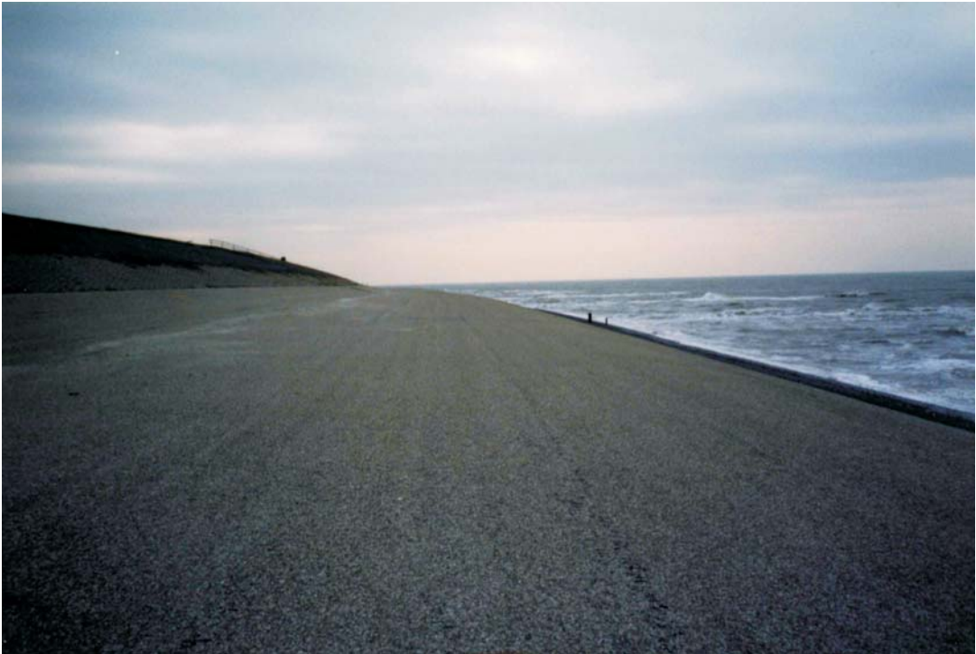
Fig. 5.16: Dike covered by asphalt (photo: SCHÜTTRUMPF)
