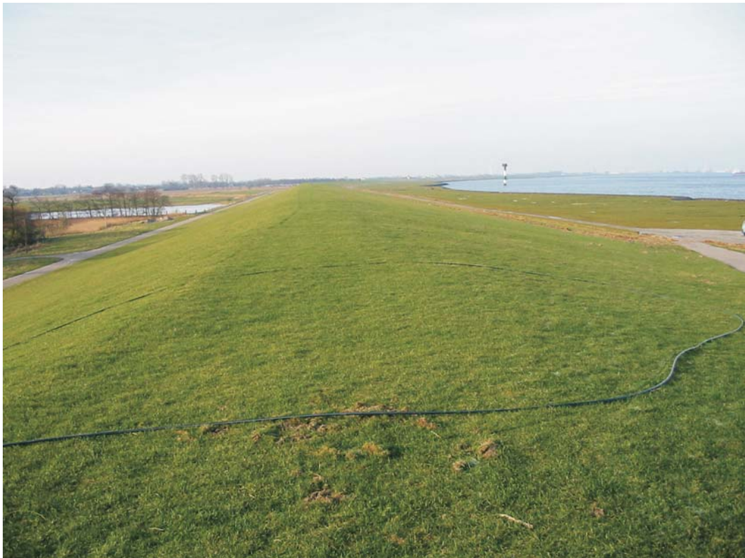
Fig. 5.15: Dike covered by grass (photo: SCHÜTTRUMPF)
