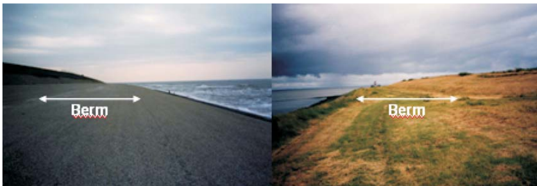
Fig. 5.28: Typical berms (photo: SCHÜTTRUMPF)
