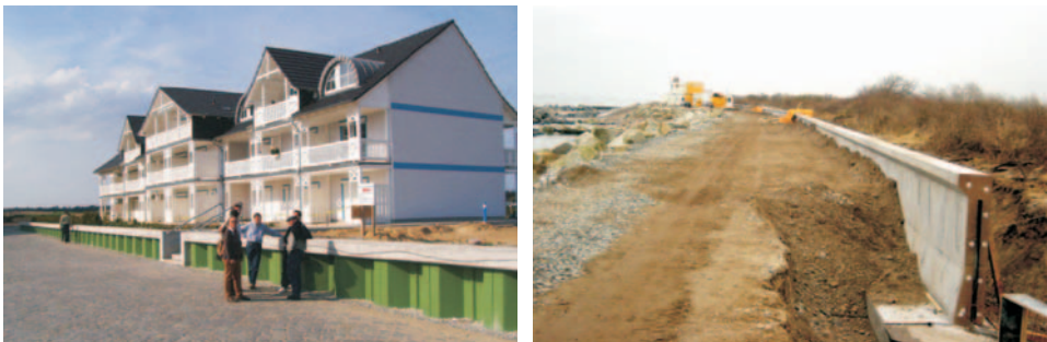
Fig. 4: Sheet pile wall with concrete cap (Karlshagen, left; length: 183 m) and cantilever retaining wall (Heiligendamm, right)
