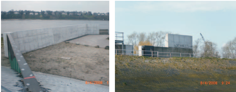
Fig. 11: Private storm surge protection in Köhlfleethafen: (left: new cantilever retaining wall; right: difference between old SPW at NN + 7.50 m and new SPW at NN + 9.30 m) (photos: HPA, 2008)
