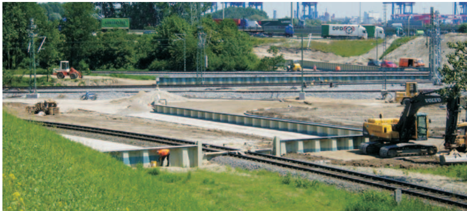
Fig. 9: Use of different protection gates (bulkhead gate in front and revolving gate, rear) at Dradenau main dike along the northern head of the port railway station “Alte Süderelbe” as part of the public storm surge protection (photo: HPA, 2006)
