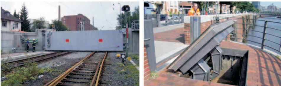
Fig. 8: Use of a flood protection lift gate (left side) and a flap gate for flood protection (right side) as part of the public storm surge protection (photos: LSBG, 2007)
