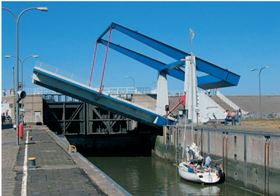
Fig. 7: Lock chamber with bascule bridge/© WSA Tönning
