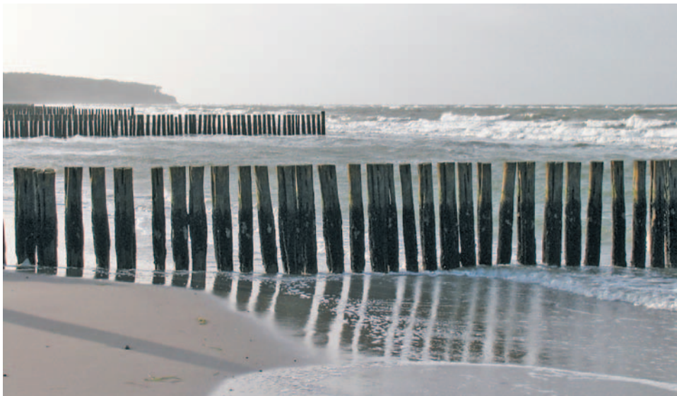
Fig. 1: Wooden single-row pile groynes at low water at the Baltic coast near Warnemünde (photo: WEICHBRODT, 2006)
