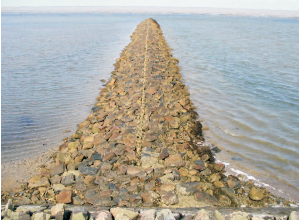
Fig. 2: Rock groyne at 'Hallig (holm) Südfall' (photo: HINRICHSSEN, 2005)
