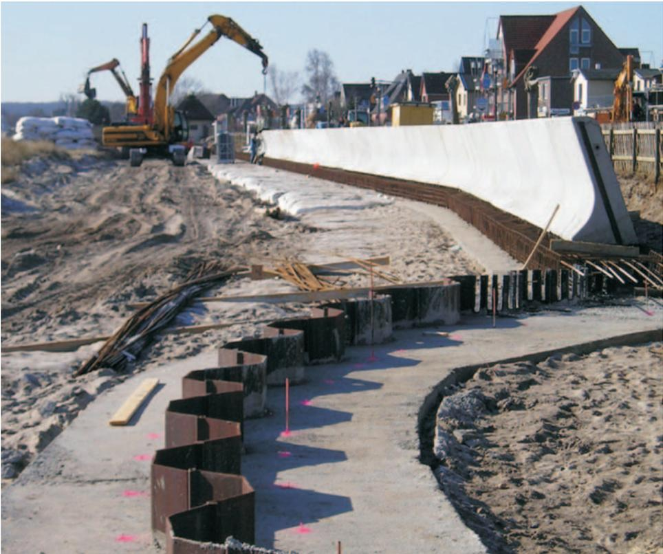
Fig. 8: Sheet pile walls mounted with concrete holms and fronted by sand containers
