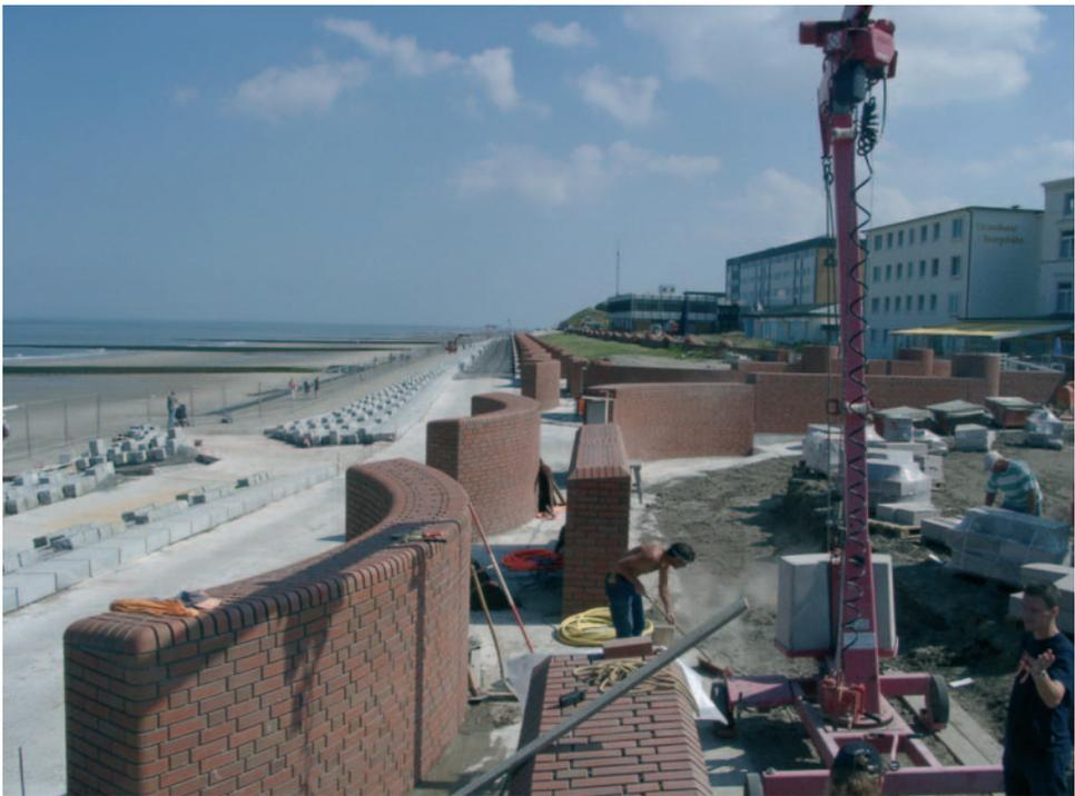
Fig. 8b: Wave run-up reduction elements at Norderney
