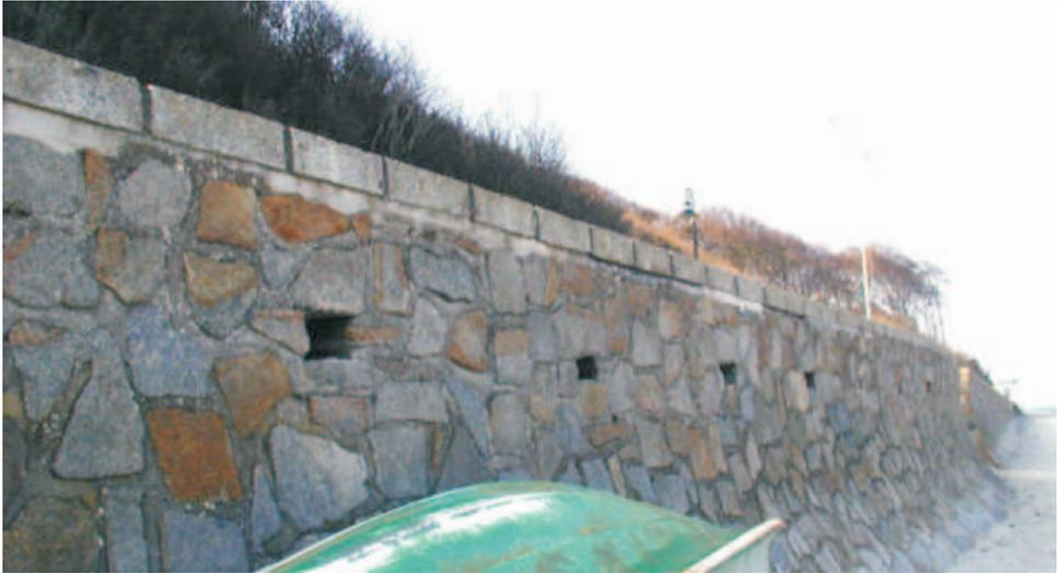
Fig. 3: Typical example of a gravity type wall in Nienhagen (Baltic Sea)
