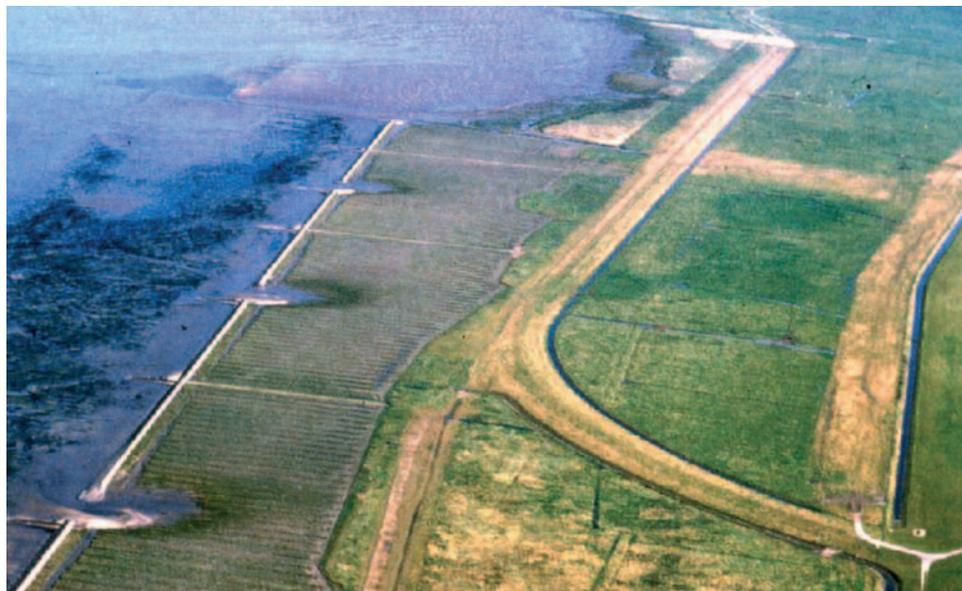
Fig. 5: Salt marshes and groyne fields in front of a primary dyke
