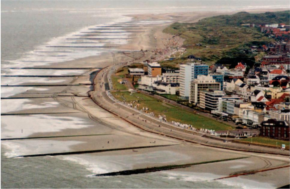
Fig. 8a: Revetment and groyne system at Norderney
