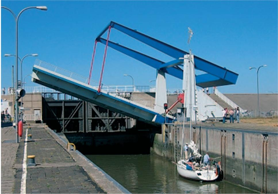
Fig. 7: Lock chamber with bascule bridge/© WSA Tönning
