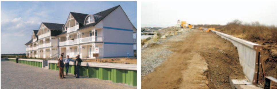
Fig. 4: Sheet pile wall with concrete cap (Karlshagen, left; length: 183 m) and cantilever retaining wall (Heiligendamm, right)
