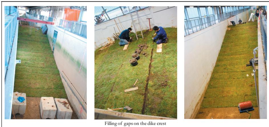
Fig. 36: Creating grass cover on the clay layer of a North Sea dike in the GWK
