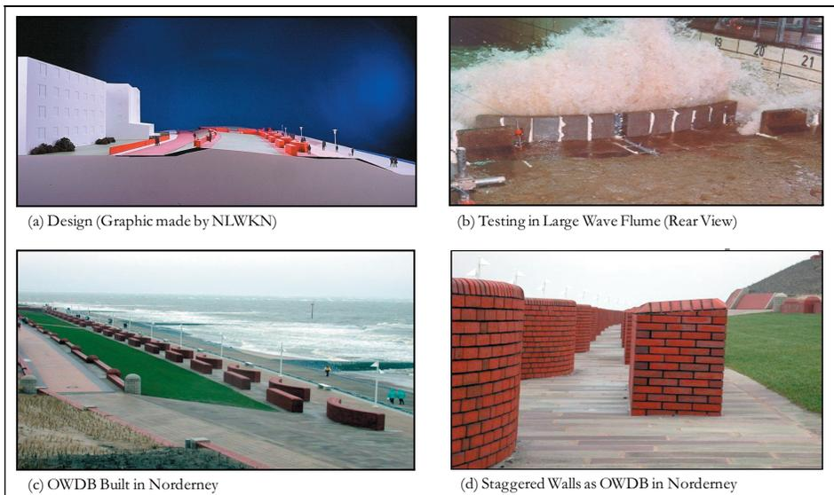
Fig. 25: Onshore Wave-Damping Barrier (OWDB)
