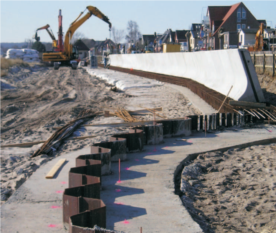
Fig. 8: Sheet pile walls mounted with concrete holms and fronted by sand containers
