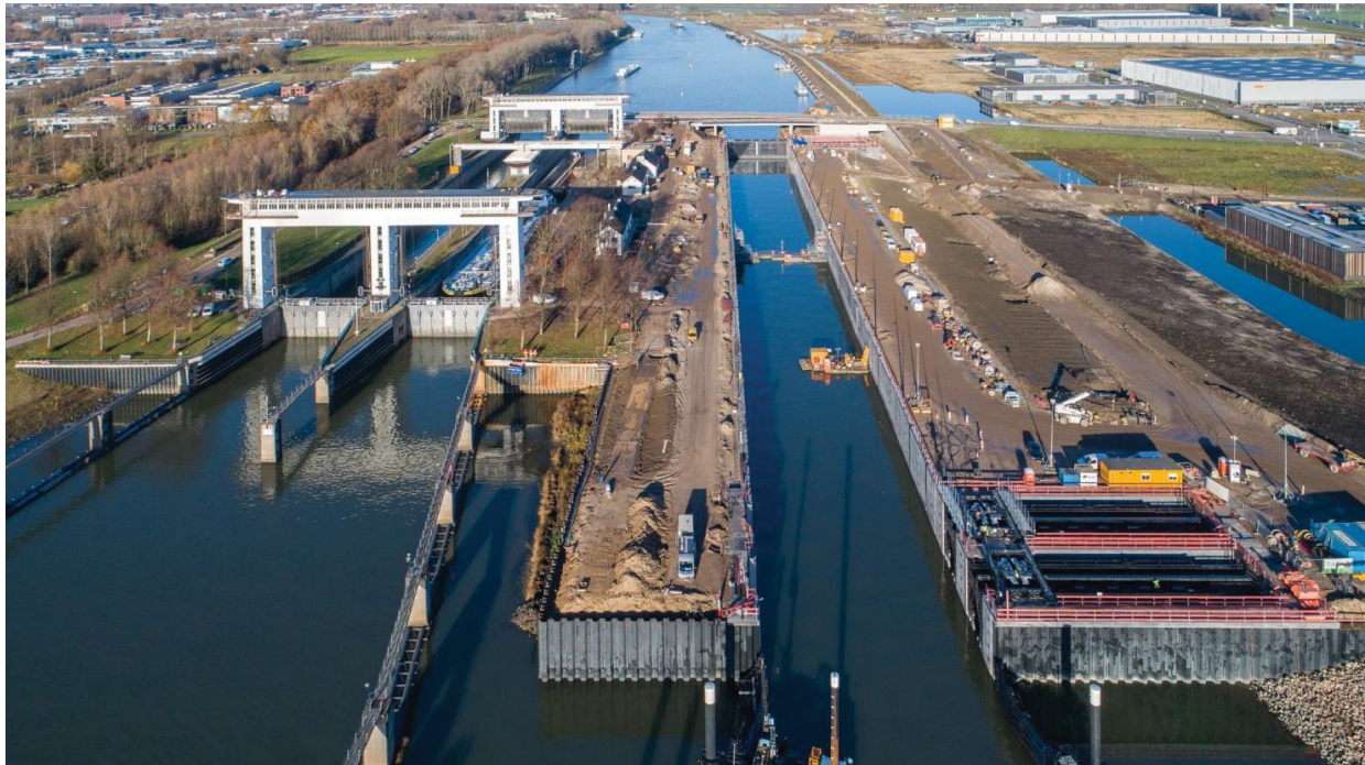
Figure 4: Overview of the construction of the new lock chamber.
