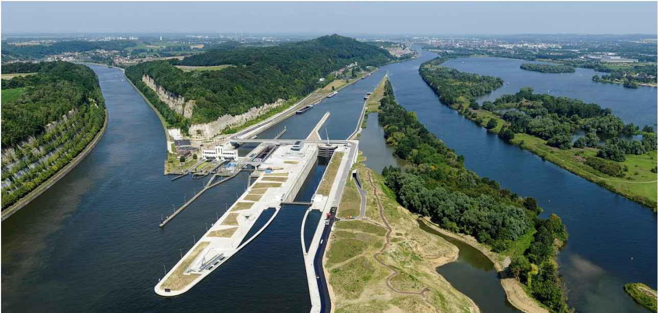
Fig.1: Lanaye Lock Complex – © JL DERU / photo-daylight.com
