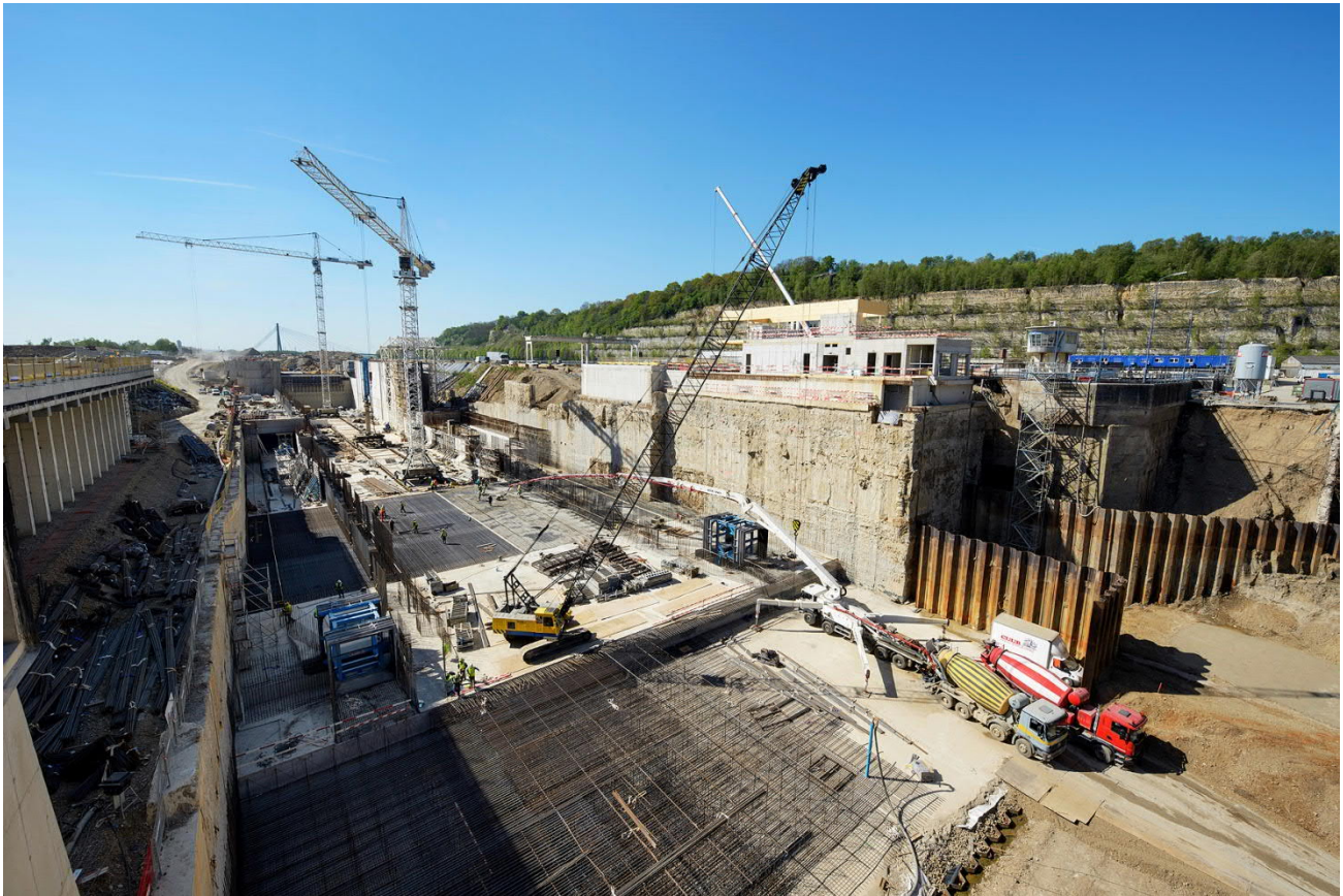
Fig.9: Construction stage of the lock chamber- © JL DERU/photo-daylight
