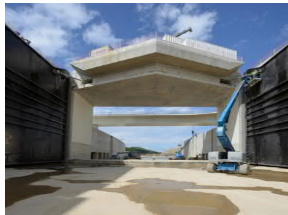
Fig.6: Downstream mitre gate – © JL DERU/photo-daylight
