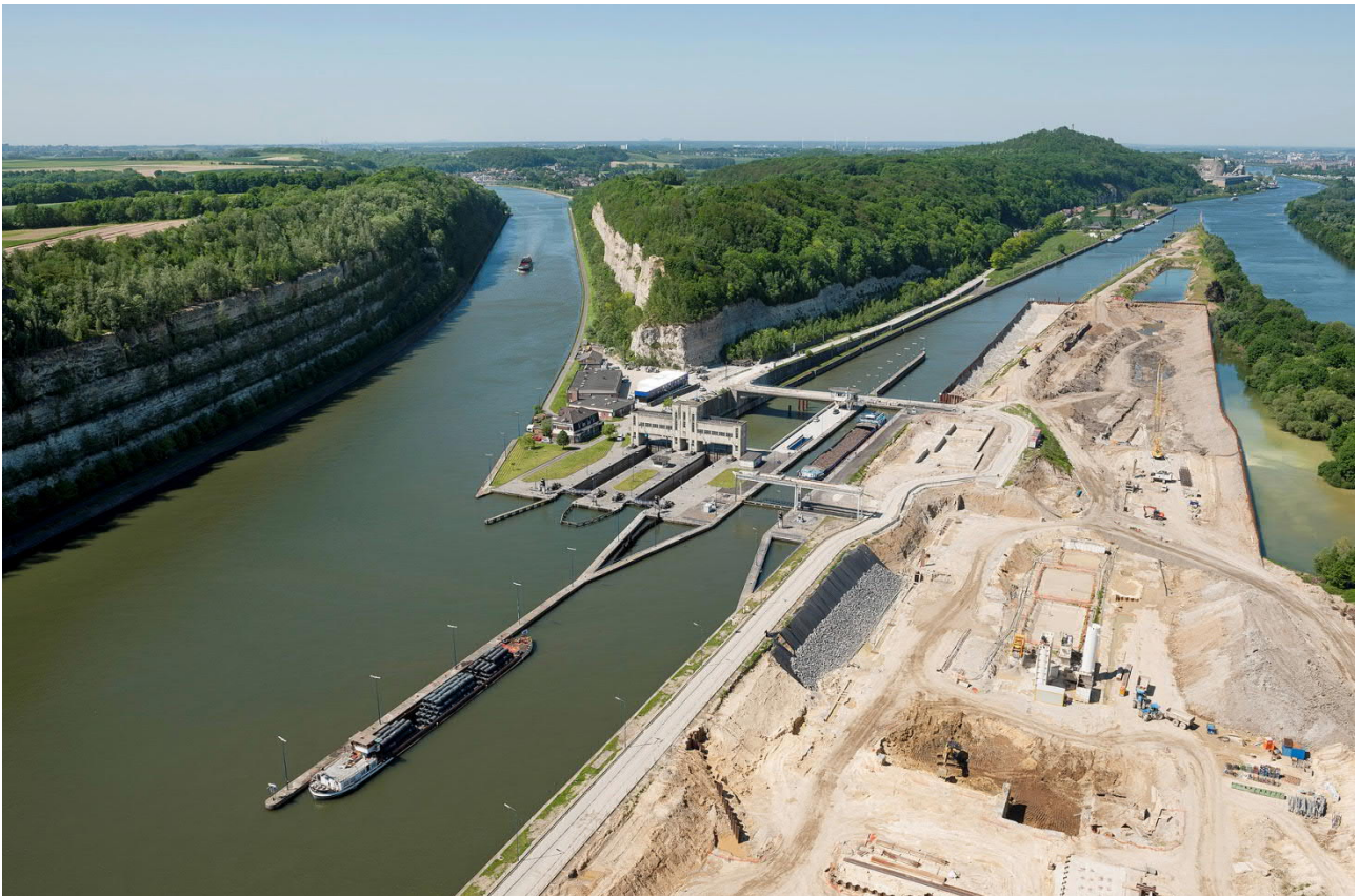
Fig.8: Overall view during excavations– © JL DERU/photo-daylight
