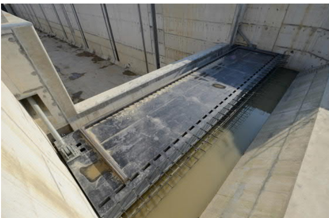
Fig.5: Upstream flap gate – © Greisch
