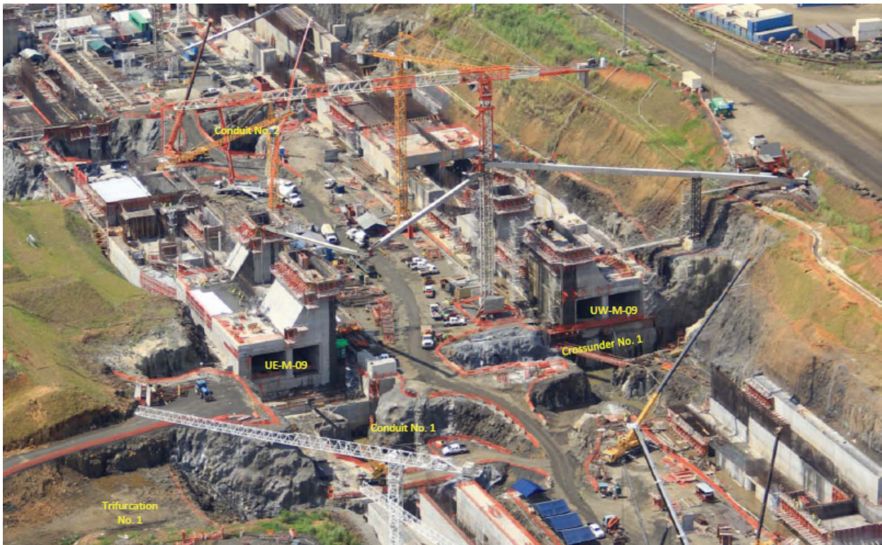
Figure 5: Construction progress of Third Set of Locks upper chamber
