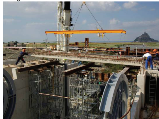
6/ sept.2007 – the works began on the promenade deck
