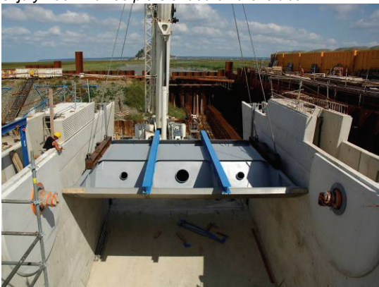
5/ aug. 2007 – installation of the first sluice gate
