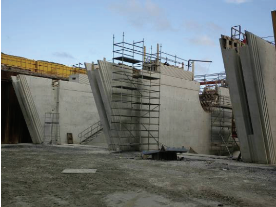
3/ july 2007 – three piers ended on the left bank
