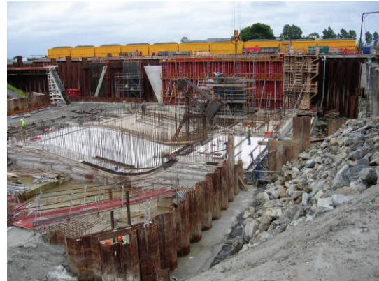
2/ may 2007 – concreting the bottom raft
