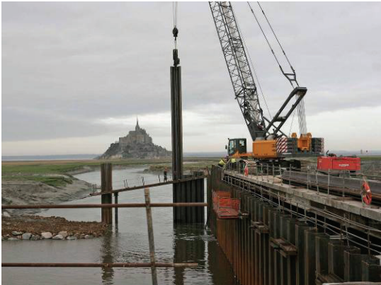
1/ dec. 2006 – construction of the cofferdam before works
