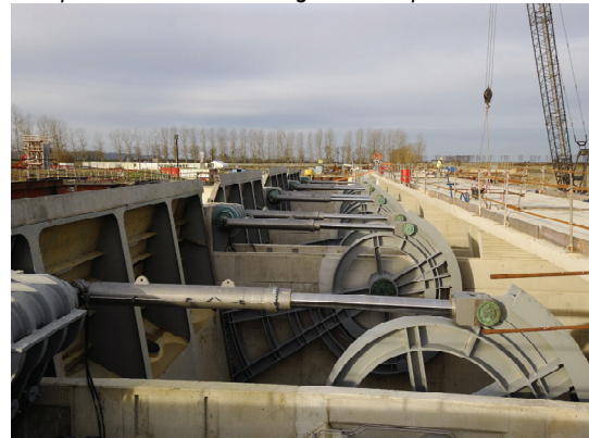
8/feb. 2008 – the gates and the jacks are assembled
