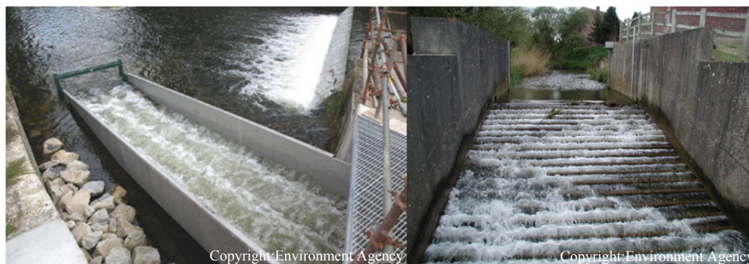
Figure 2: A Larinier fish pass on a flow gauging weir (left) built to ISO 26906:2009 and Low Cost Baffles (right) designed to ISO/AWI TR 19234
