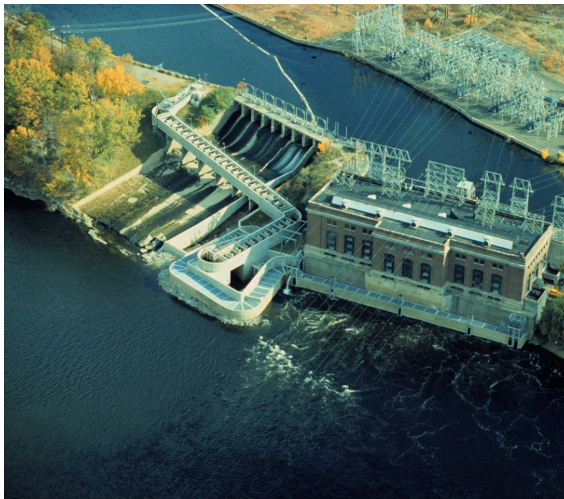
Figure 3: Cabot fishway, RKm 194 on the Connecticut River, Massachusetts USA. Constructed in 1980, this fishway has probably never passed shad effectively.
