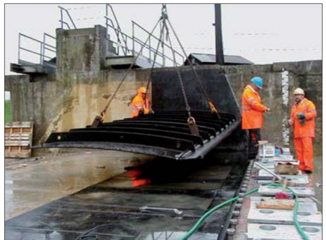
Figure 5: Placing a gate on top of a bladder
