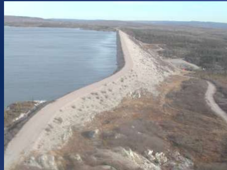
Existing structures (after seepage detection investigations?)
